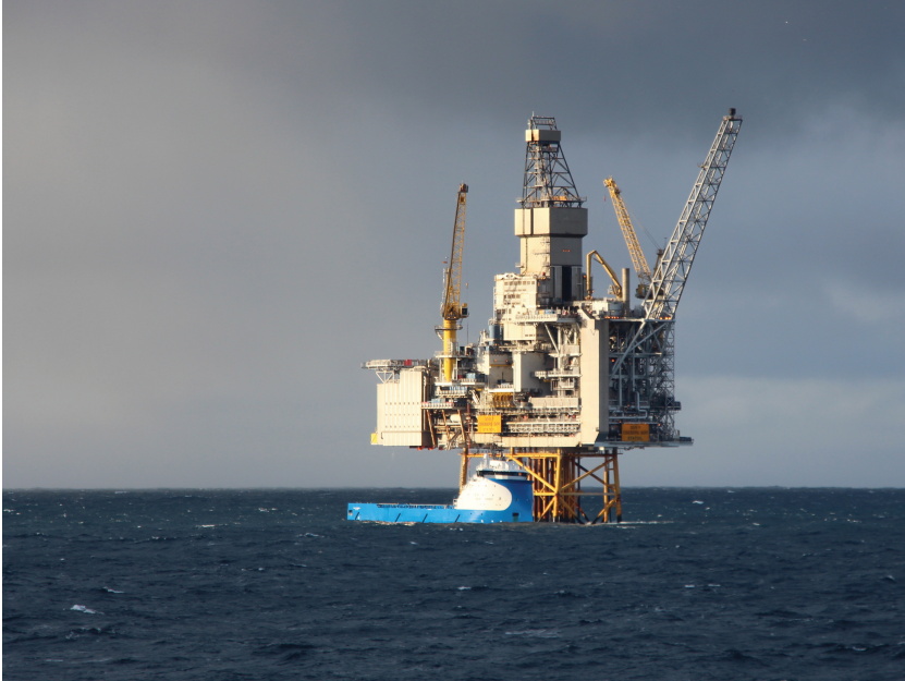
Figure 2: Platform supply vessel next to a rig in the North Sea. (Photo: Ulstein Group)
