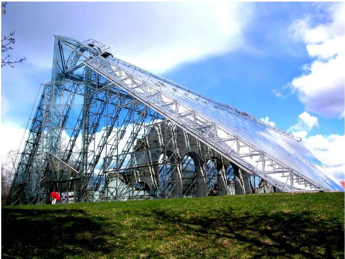
Illustration 81: Glass and steel construction over the medieval Domkirke ruins, Hamar by Sverre Fehn.
