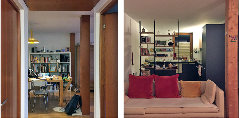
Figure 2.13 Constructive grid of the column-based load-bearing system at Ölbündt – increasing flexibility regarding the placement of walls, limiting furnishing options.
