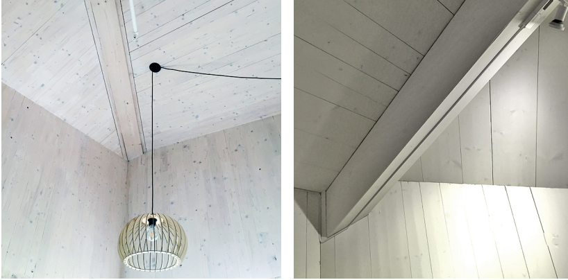
Figure 2.7 Beam meeting irregular angles at a) Ulsholtveien and b) Skadbergbakken.
