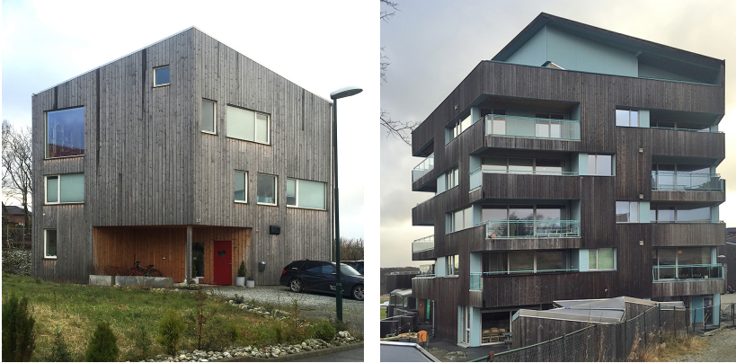
Figure 3.8 Two ways of handling colour changes in parts with different weather exposure at Skadbergbakken, using a) wood that will retain its original colour where not exposed to sun and rain or b) applying coloured trespas.
