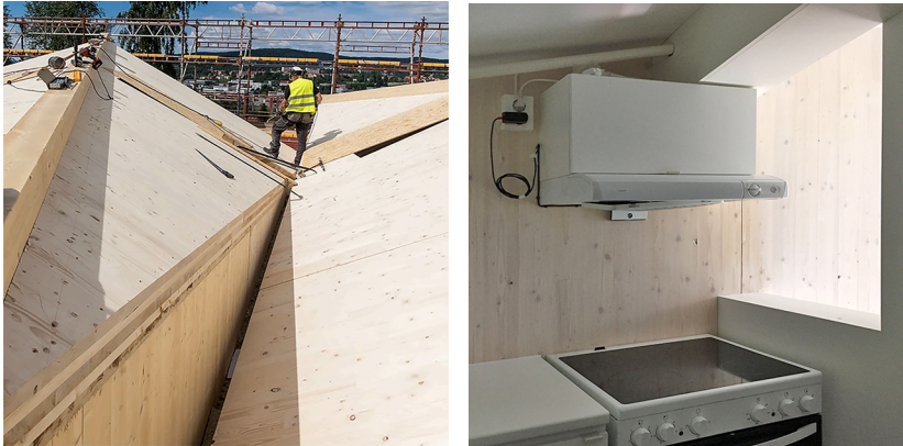
Figure 2.4 a) Double CLT wall separating two units, Ulsholtveien, 2017, Haugen/Zohar. Photo: hza.no. b) Cooktop against exposed, oiled CLT wall at Ulsholtveien.
