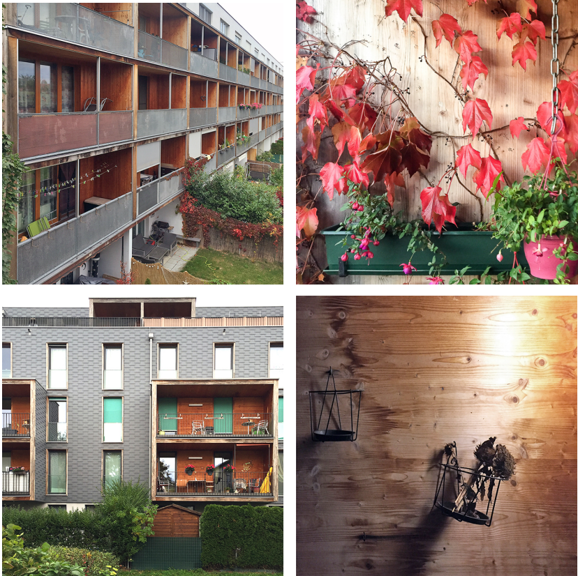
Figure 3.7 above: Loggia wall turning silvery grey at Spöttlgasse (accepted) and below: Uneven weathering in the top floor loggia at Mühlweg (B) (disliked)
