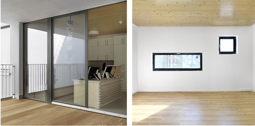
Figure 2.3 Permanent wooden formwork in the ceiling of c13, Kaden+Lager, 2014. Photo: Bernd Borchart
