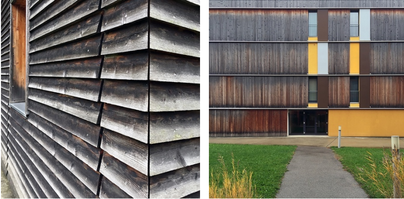
Figure 3.4 a) Ölzbündt is ageing together with its first inhabitants. Greying surface and long-lasting precision 20 years after completion. b) Uneven weather exposure of the façade at Mühlweg (A). Acceptance for both.
