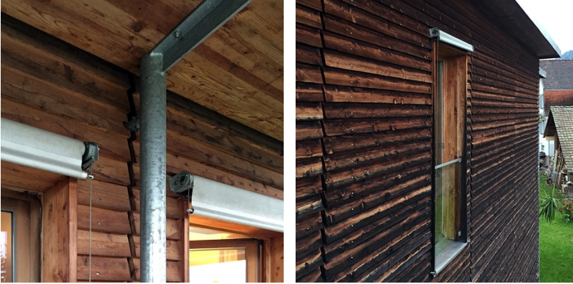
Figure 3.6 Two adjacent façade areas at Ölbündt: a) Little colour change in protected areas, and b) unevenly weathering horizontal boards where exposed to sun and rain. Every panel weathers differently, depending on its angle and position on the façade.
