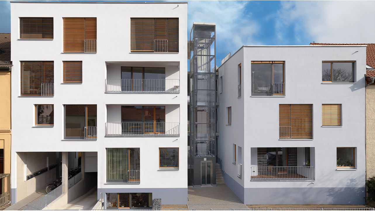
Figure 1.42 sw40 2011, Architect: Kaden Klingbeil Architekten, Photo: Bernd Borchardt
