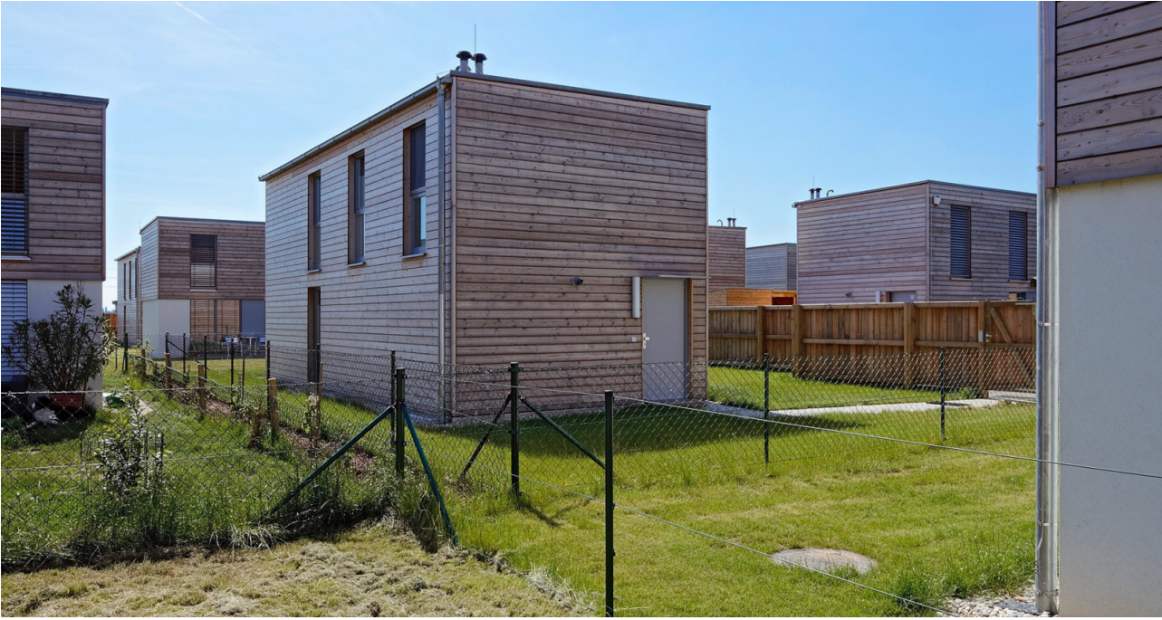
Figure 1.28 Lobaugasse 2009, Architect: Dietrich I Untertrifaller, Photo: Bruno Klomfar
