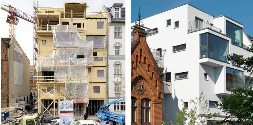
Figure 2.1 Perforated façade combined with window placement in gaps between constructive parts in C13, Berlin, 2014, Kaden+Lager. Photos: Bernd Borchart
