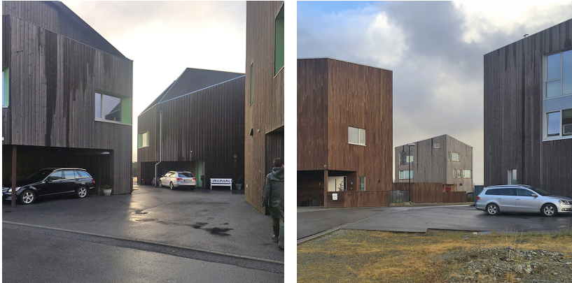
Figure 3.5 a) Dark and uneven surfaces, and b) individualizing colour changes at Skadbergbakken
