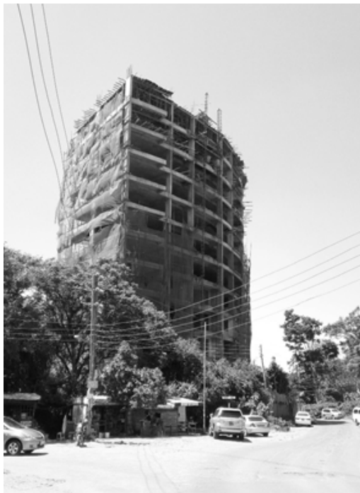
FIGURE 4 High-rise apartment block under construction in Kileleshwa, Nairobi Source: Author 2018
