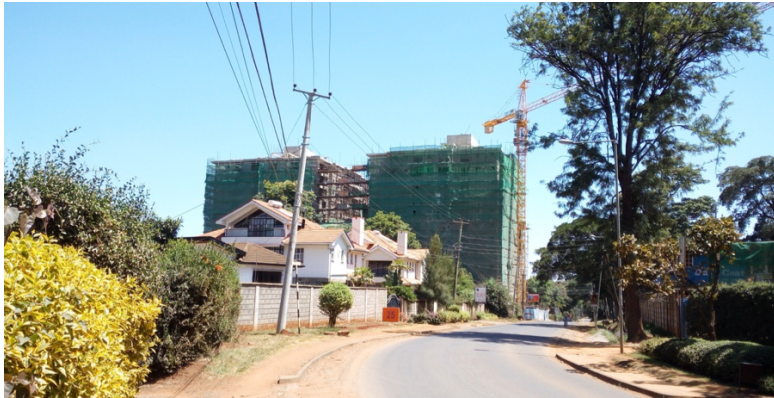
Figure 4.22 Kileleshwa: High-rise apartment blocks under construction. (Author, 2018)
