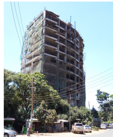
FIGURE 20 Kileleshwa: A high-rise apartment block under construction Source: Author 2018
