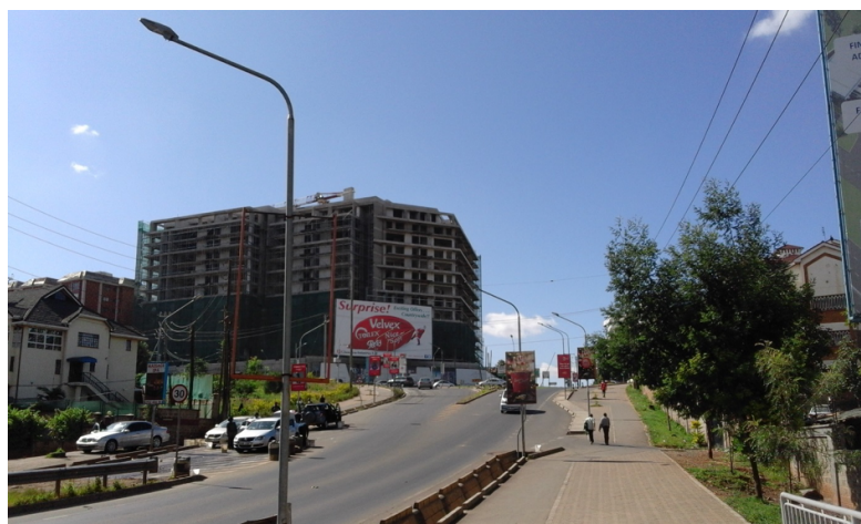
Figure 4.12 A high-rise apartment block under construction in Kileleshwa, Nairobi. (Author, 2016)
