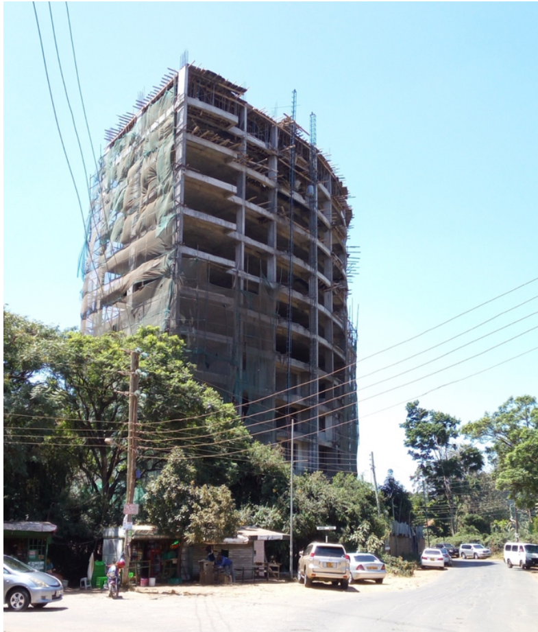
Figure 4.23 Kileleshwa: A high-rise apartment block under construction. (Author, 2018)
