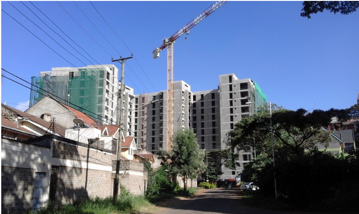
Figure 1: A high-rise apartment under construction in Kileleshwa neighbourhood, Nairobi (Source Author, 2015)
