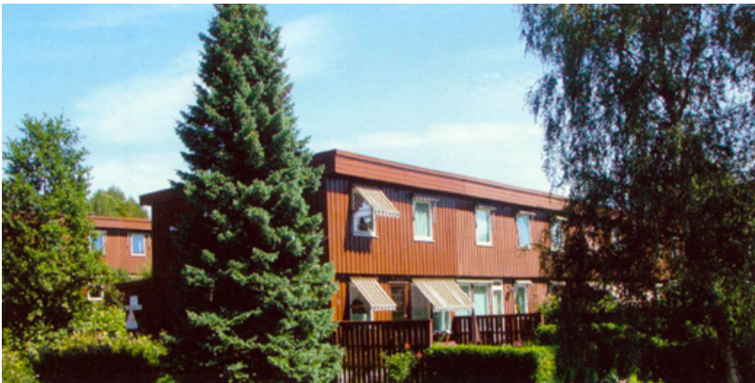
Fig. 15. Among Moelven main products were prefabricated row-houses in timber. Above, a housing development in Øvre Høybråten Borettslag. Below, a project in Stovner. From OBOS: hus og hjem i 75 år .
