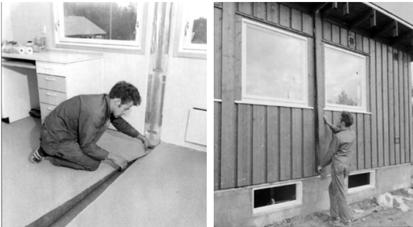
Fig. 18. On-site finish works. Photos by Fotohuset, Hamar. N-21797-4, Hedmark museum photo archive.
