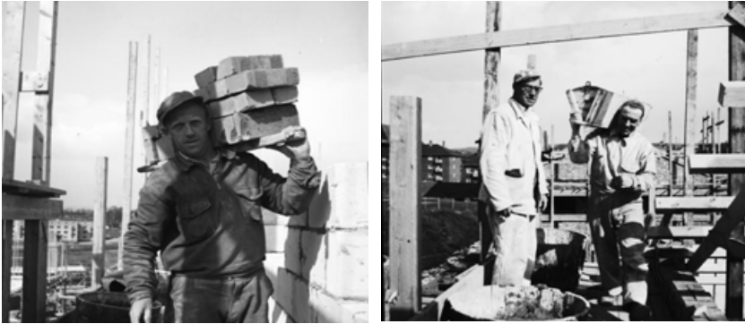
Fig. 17. Construction work in Oslo, as captured by photographers of Henriksen & Steen, 1956. Even on the larger construction projects—multi-storey housing buildings—labour was mostly performed manually, without the use of machines or building cranes. National Library photographic archive, public domain.
