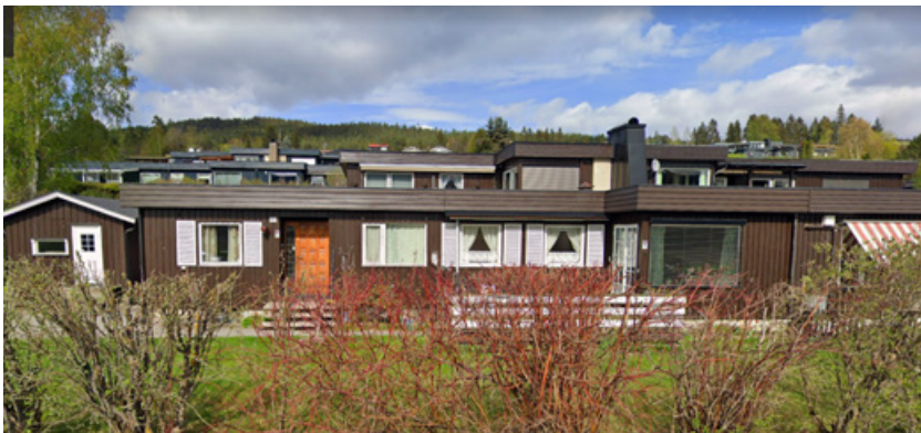
Fig. 16. Nittedal housing project developed by Yugoslavian architect Trifunovic specifically for slanted terrain. Above, project drawing and photograph from newspapers, 1966. Below, contemporary google maps image.
