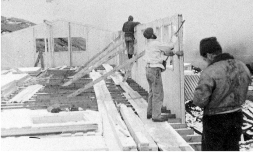
Fig. 17. Moelven element assembly on site. Newspaper clippings, 1966-1970.
