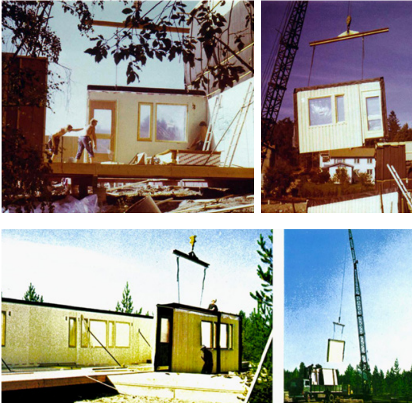
Fig. 10. On-site Moelven element assembly. Photographs from https://munkerudsletta.no/?p=12047 , accessed March 8, 2022. Below, Raufoss housing, from Moelven 1899-1999 .
