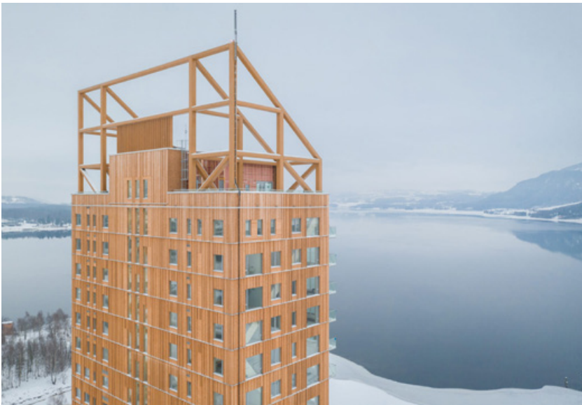
Fig. 35. Moelven Mjostårnet completed in 2019 with all load-bearing elements made in Moelven laminated timber. Photo by Woodify, https://www.woodify.no/mjostarnet-brumunddal/ , accessed August 8, 2020.
