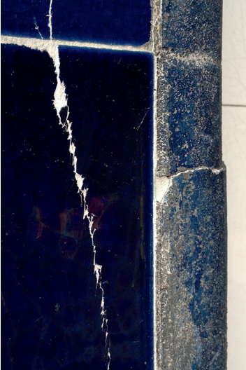
Fig. 17 Existing tiles from the original butcher's shop
