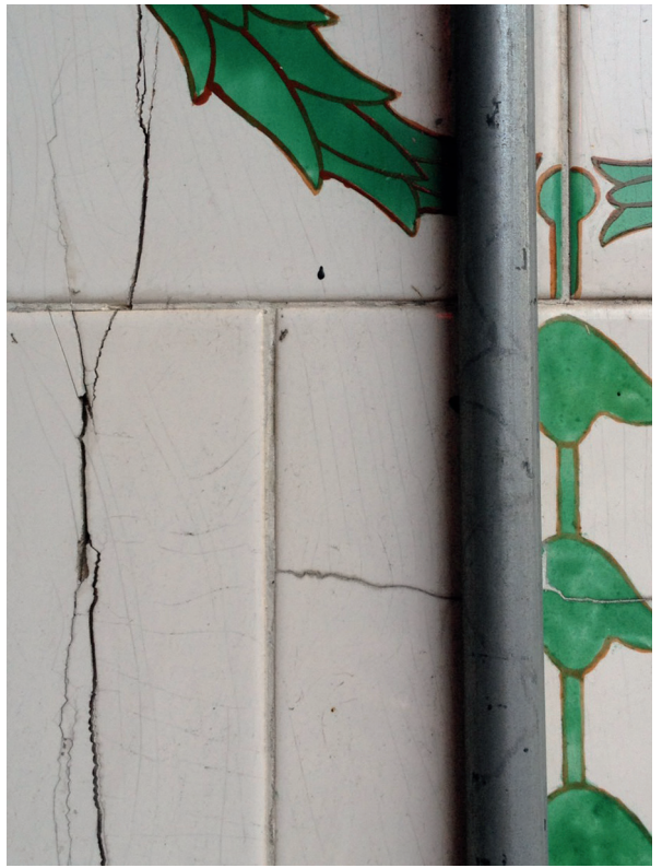
Fig. 18 Existing tiles from the original butcher's shop
