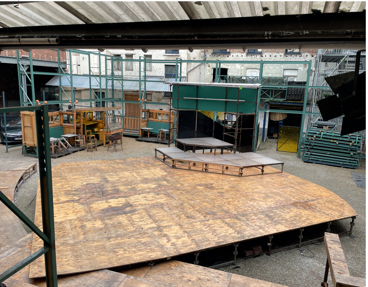
Fig. 109 Transportable wooden stage construction by Decoratelier at its courtyard
