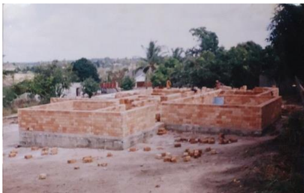
Figure 3.36: Interlocking soil stabilized blockwork under way.
