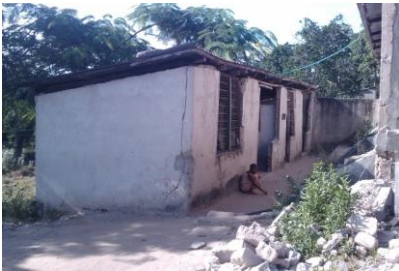
Figure 3.44: The structure used to run the elementary School.
