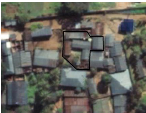
Figure 3.40: The Satellite image indicating the nature of building organization of the cluster including Mr. Goza's Property.
