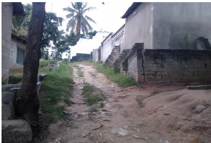
Figure 5.10: Roads provided are usually narrow as each individual developer attempts to maximize the utilization of his plot.
