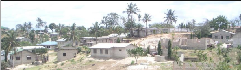
Figure 3.26: Uncoordinated developments require certain negotiations and collaboration among individual developers to generate a holistic continuity that safeguards collective interests.
