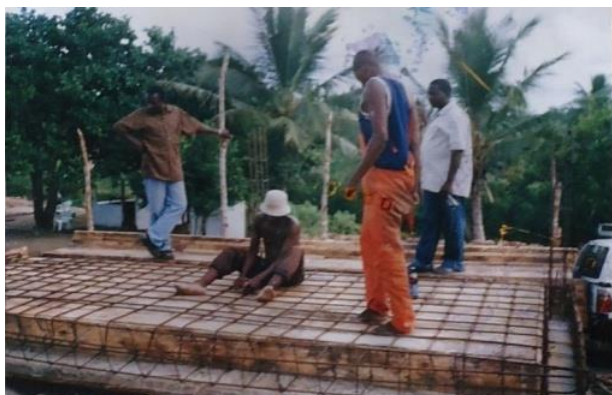
Figure 3.33: Steel fixing in progress.
