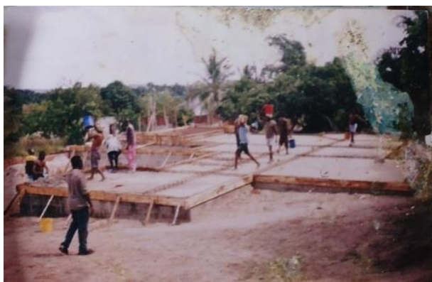
Figure 3.35: Conveying and pouring concrete into the foundations.
