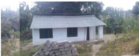
Figure 3.29: Mr Edgar’s house is made of wattle and mud walls which were smooth finished and whitewashed.
