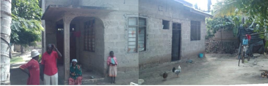
Figure 3.10: Mrs Amina's House built to the design and size desired.
