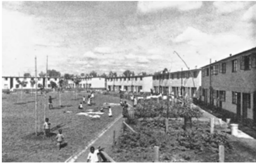
Figure 2.3 The Ofafa Jericho social housing scheme. According to McVicar the design was reminiscent of “prison-like structures” (1969, 57).
