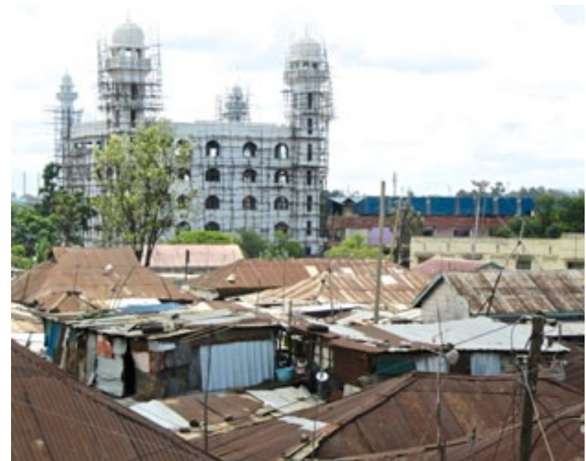
Figure 8.1 Pumwani Riyadhha Mosque under construction in 2012 (author).
