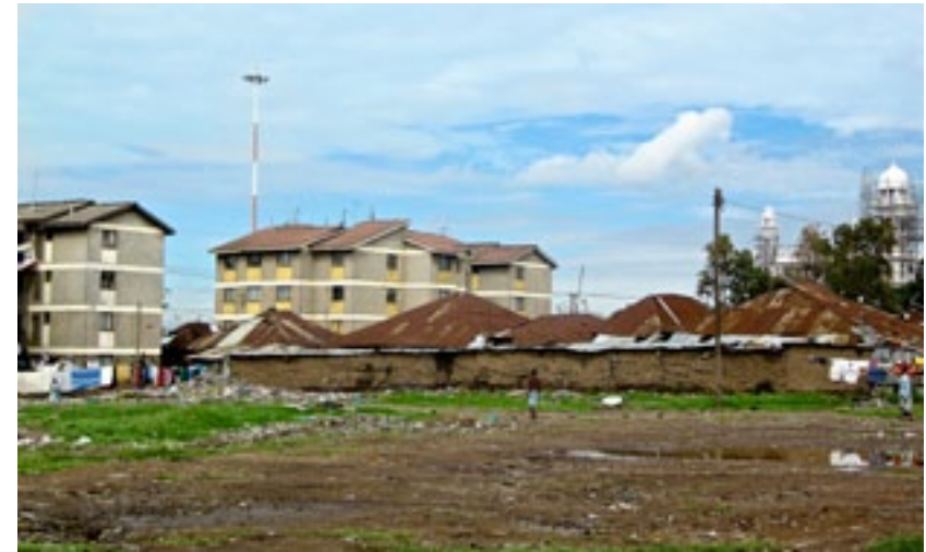
Figure 6.4 Soon to be demolished (?) Majengo houses in Bash, surrounded by the new Highrise flats (author).
