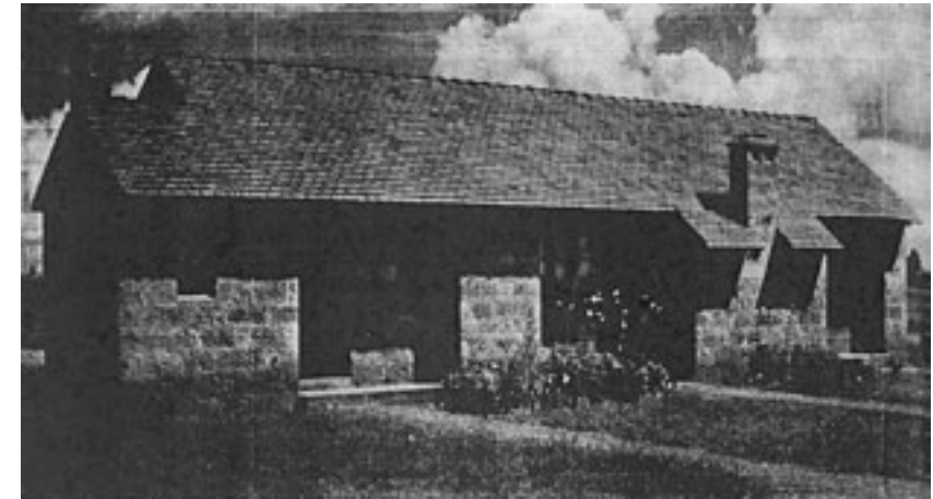
Figure 2.1 Salubrious family housing in Starehe, from Ogilvie (1946).
