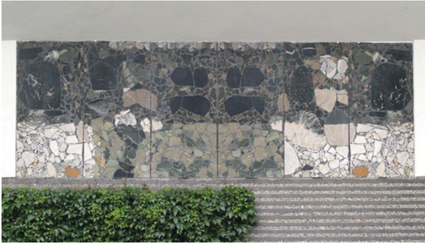
Figure 42. Conglo-betong in the façade of the High-rise annex.
