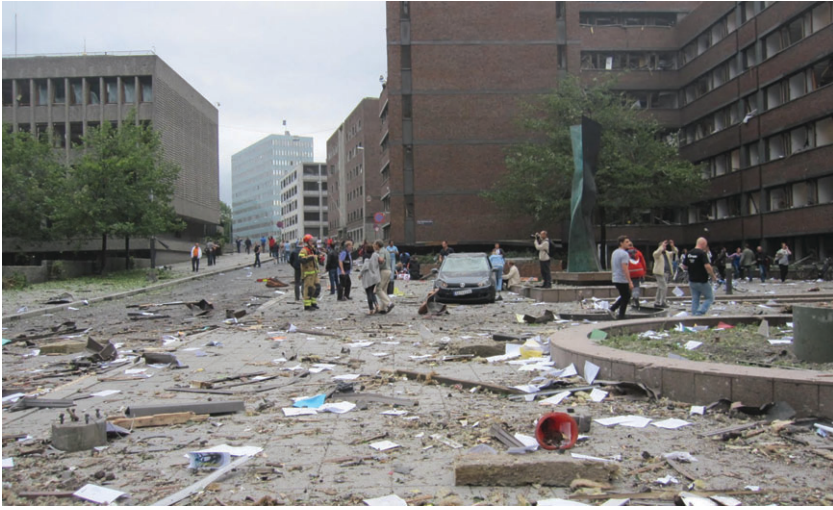
Figure 40. Grubbegata Street after the explosion. The Y block to the left and the S block to the right.
