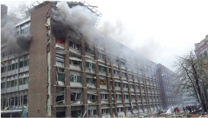
Figure 3. The R4 after the explosion, seen from Grubbegata.
