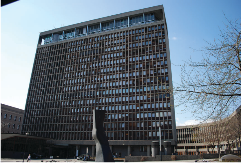
Figure 10. The High-rise seen from Einar Gerhardsens plass. 2009.
