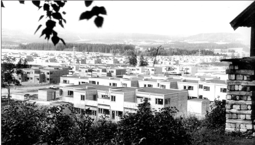
23: Skjetten Town, Nils-Ole Lund with Resen, Throne-Holst and Hultberg, 1967–73 (Photo: Taken from Arkitekten 10–11/1973).
