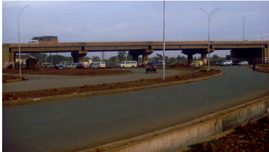
Plate 5.1: A picture showing the overpass at Roysambu along the Thika Superhighway after the transformations. (Source: M. S. Kimunyu)
