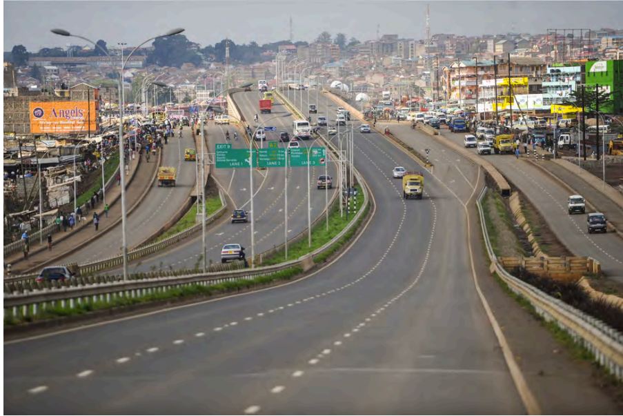
Plate 5.6: A view of the Githurai roundabout from the Kahawa drift showing the new physical elements of the 10-lane highway at this intersection. The 6 lanes of the expressway serve through traffic and are elevated above the roundabout in the background. Two-way service roads accessed from exits from the main highway connect the local area. (Source: fountainnews.co.ke)
