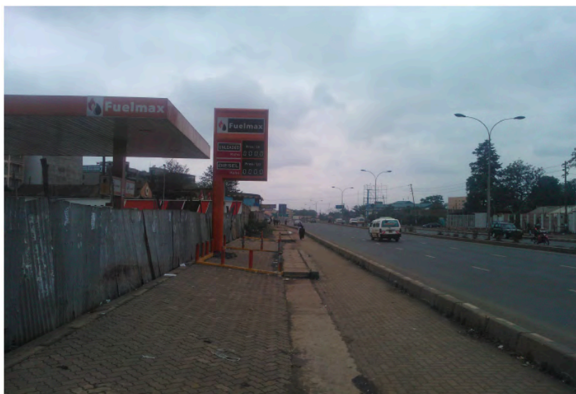
Plate 4.2: A stretch along Murang'a Road showing an abandoned filling station after access was restricted by a kerb after the transformation of the highway. (Source: Author)
