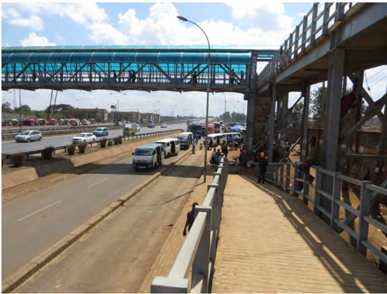
Plate 5.9: The Roysambu bus stop and the Roysambu footbridge along the Thika Superhighway after the transformations. Such footbridges serve all other non-motorised transportation modes including domestic animals. (Source: Author)
