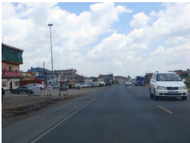
Plate 5.45: Buildings along the Eastern Bypass at Utawala Township after the transformations. The township has grown by a process of rapid accretion after the opening of the highway. (Source: Author)
