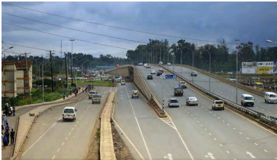
Plate 5.7: A view of the roundabout at Roysambu from the Roysambu footbridge showing the new physical elements of the highway and service roads at this intersection. (Source: Z. Mutunga)
