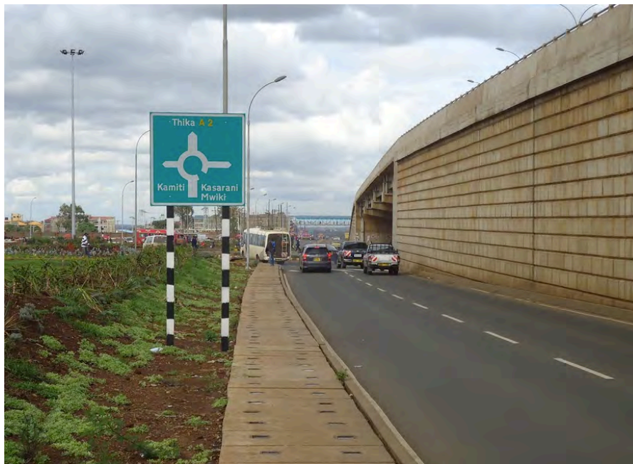
Plate 5.2: A picture showing the retaining wall supporting the expressway overpass at Roysambu along the Thika Superhighway after the transformations. The prior visual connection between the opposite sides of the highway is lost. (Source: Daniel Thuku)
