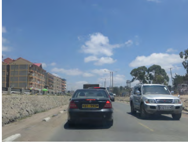
Plate 5.53: A section of the highway showing the separation of pedestrian and vehicular traffic at Kitengela Township after the transformations. The crash barrier to the right bifurcates the township. (Source: Author)
