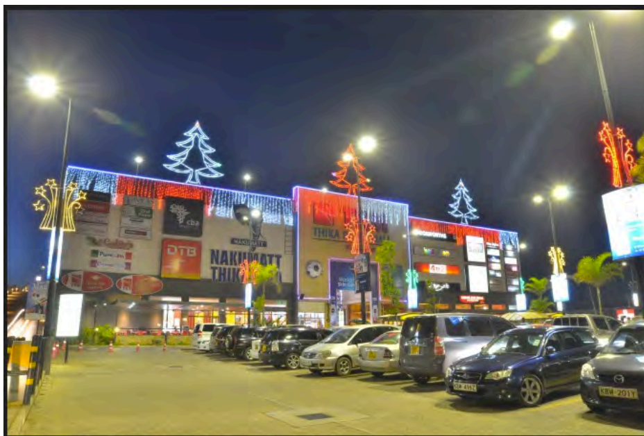
Plate 4.5: The façade of the Thika Road Mall facing the Thika Superhighway. Abutting the other faces of the mall are high-rise residential tenement buildings in an informal settlement from which the mall is insulated by 3-metres high fences, a deliberate lack of openings and the service zones. The roof of the mall, from which the informal highrise apartments around the mall would be visible, serves as car parking thus completing the "hermetic seal." (Source: www.trm.co.ke ; accessed on 21 st May, 2015)
