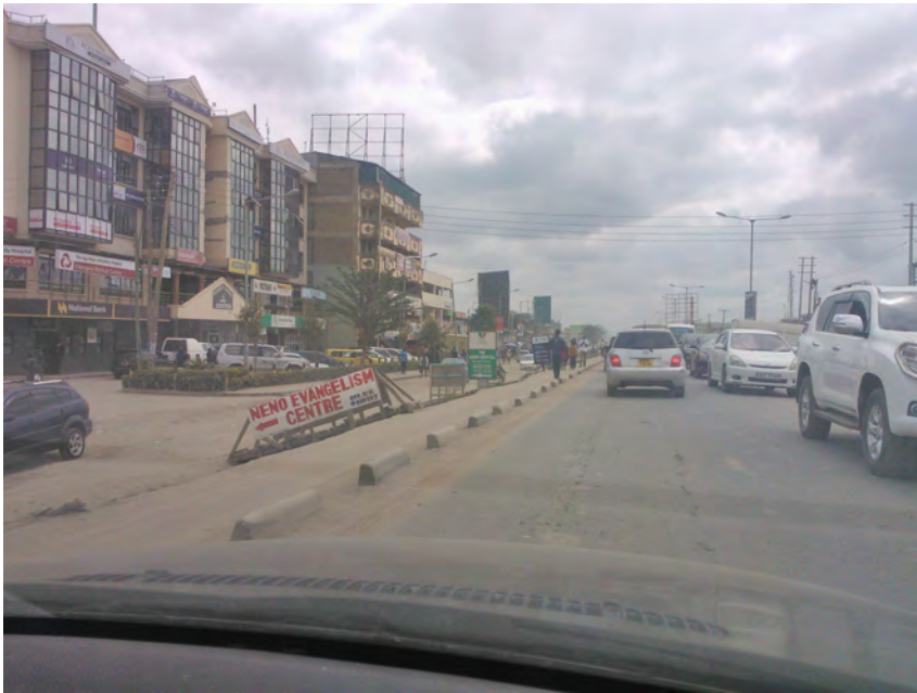
Plates 5.61 (above) and 5.62 (below): A series of makeshift bridges made across the drainage channel at the township so as to reconnect social spaces that transcend the highway. (Source: Author)
