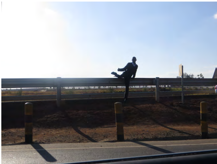
Plate 5.42: A pedestrian hops over a crash barrier at City Cabanas along the Airport North Road after the transformations. (Source: Author)
