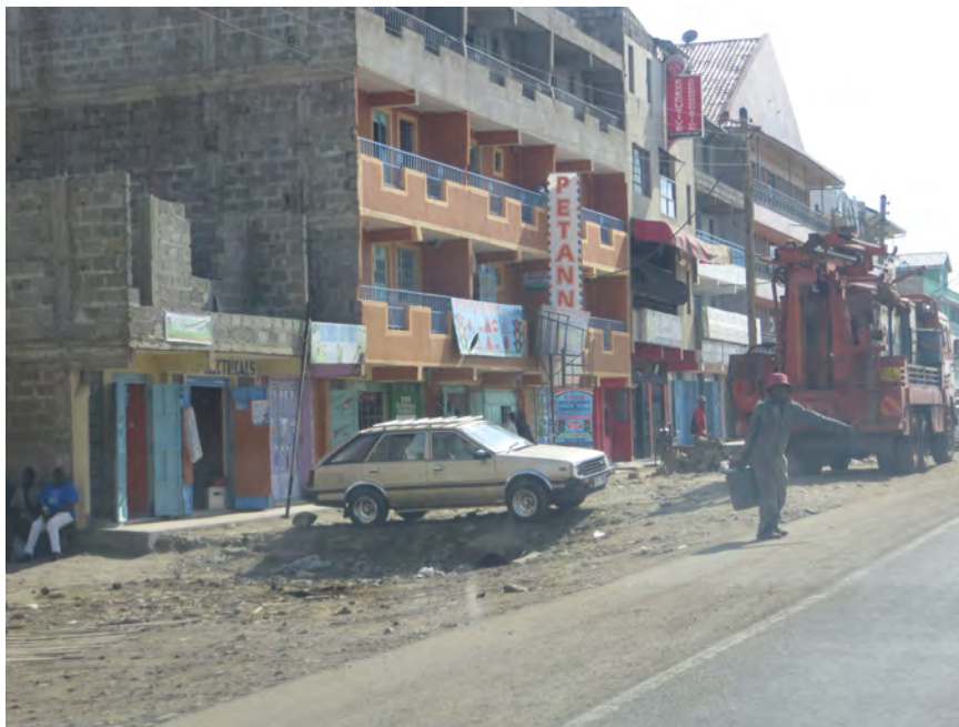
Plate 5.47: Incremental building construction along the highway at Utawala Township after the transformations. (Source: Susan Njeri Omollo)
