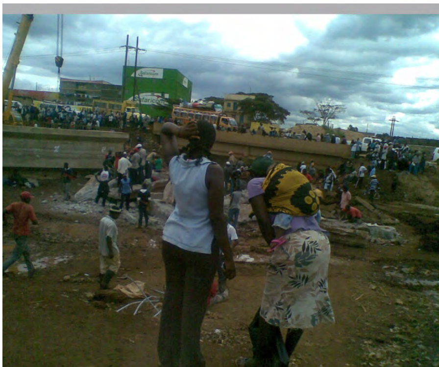
Plate 5.3: Crowds gather near the Thika Highway at Githurai On 5 th November, 2008 to collect recyclable waste (such as rebar and stone) after the demolitions of structures and buildings to make way for the 10-lane expressway. (Source: The Daily Nation, 11 th September, 2010)
