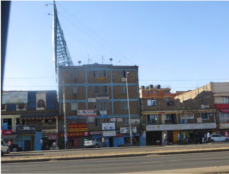
Plate 5.43: A picture of section of the highway through Embakasi along the Airport North Road after the transformations. The highway/building interface is 3 metres with no provision for parking. (Source: Author)
