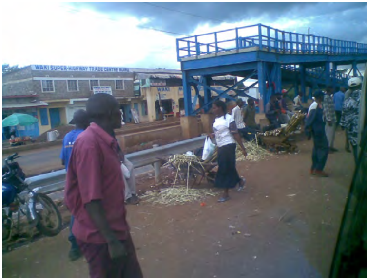
Plate 1.5: A scene of the bus stop and footbridge at Ruiru. This is an example of how displacement, reinvasion and adaptation by informal activities occur within road space along the Thika Superhighway. (Source: Author)
