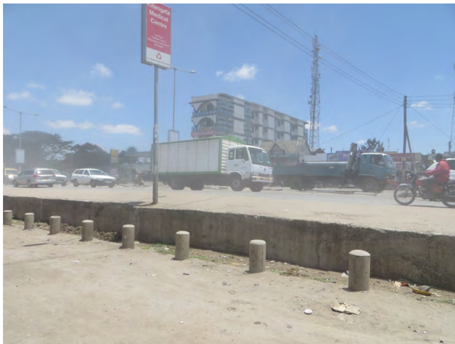
Plate 5.52: A section of the highway through Kitengela Township after the transformations. Though the road construction conformed to the slope across the township no linkages were constructed to bridge the two sides of the main shopping street. (Source: Susan Njeri Omollo)
