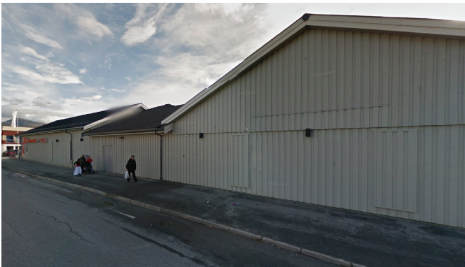
Wall between waterfront and Fauske
