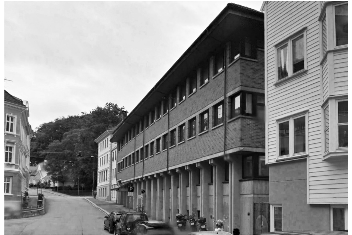
IMR office addition
