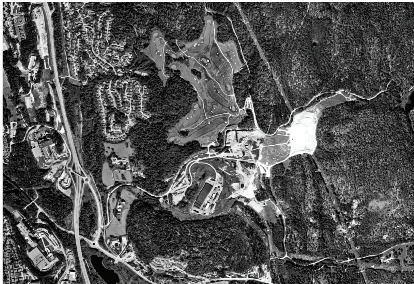
Original site situation
