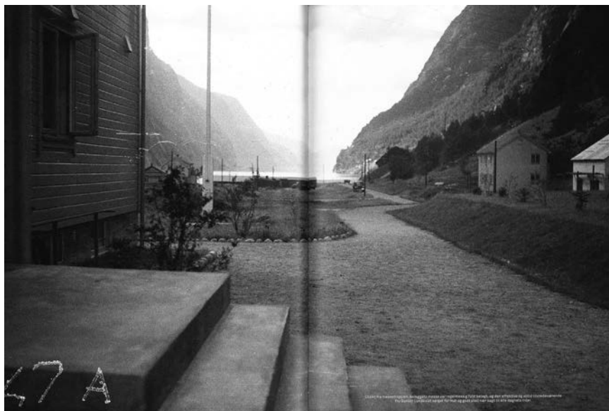
View from the entrance of the "messe", a building serving as dining and living room for the workers.
