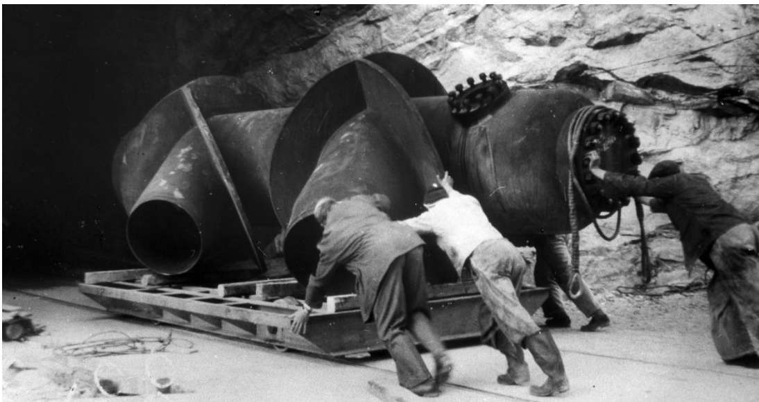
Rails was installed to help place the parts for the machines.
