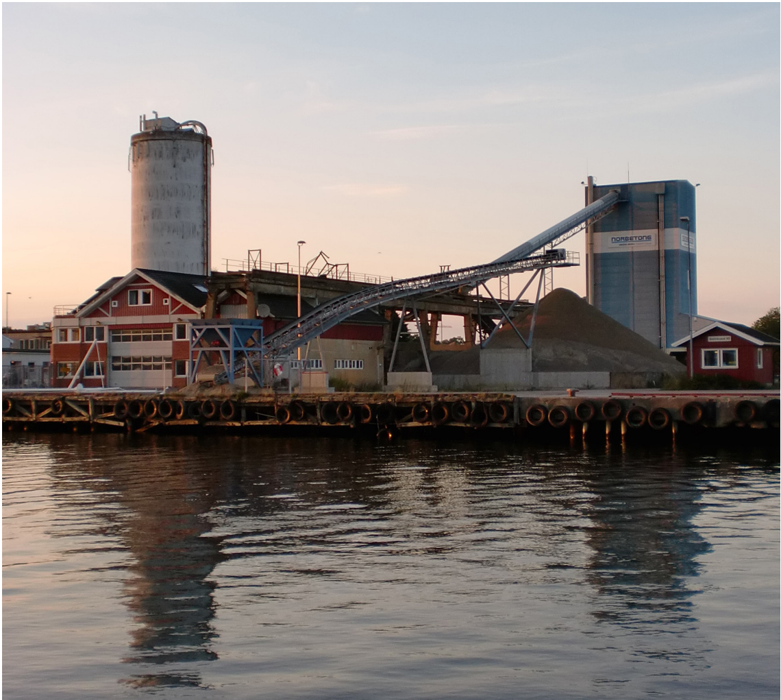
Foto, Stensarmen , Concrete factory
