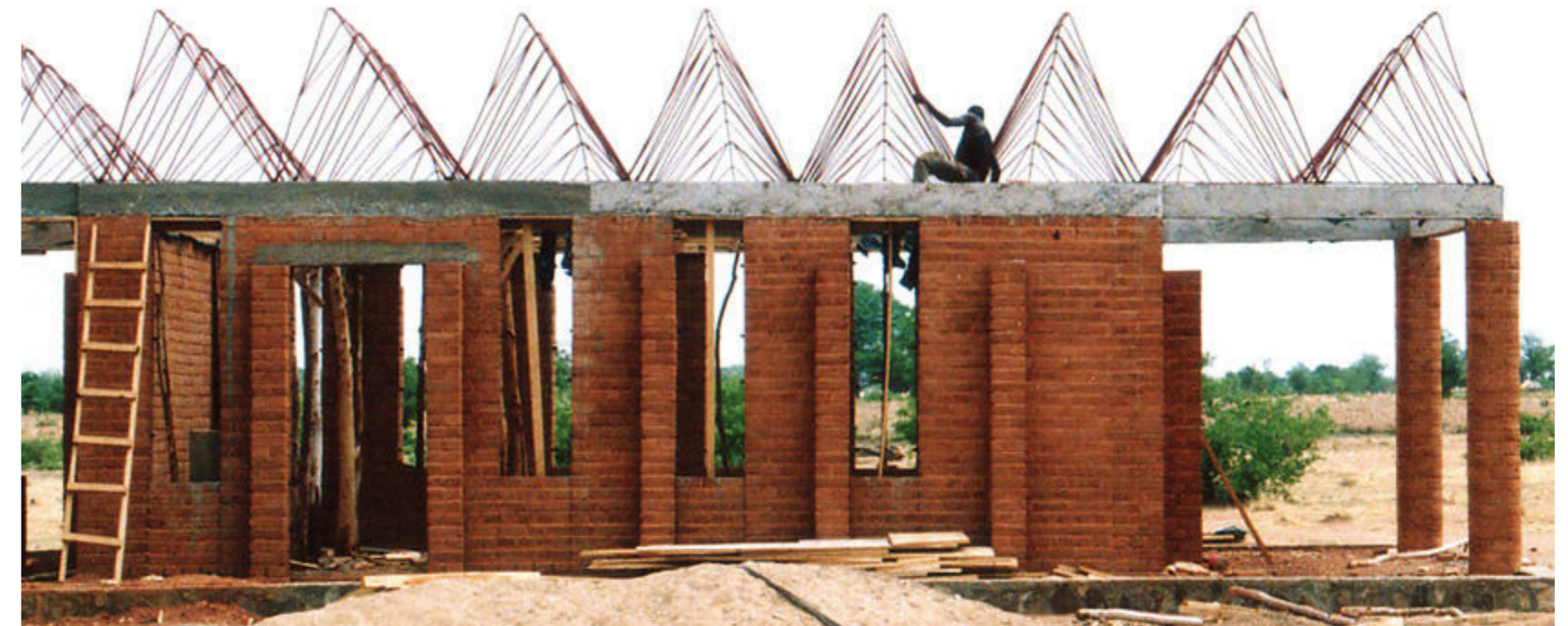
Figure 21. Gando Primary School by Francis Kéré, during construction (Moma, 2003)
