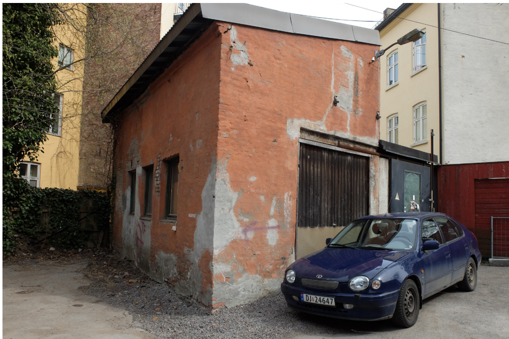
Brick shed in backyard Akersveien 20
