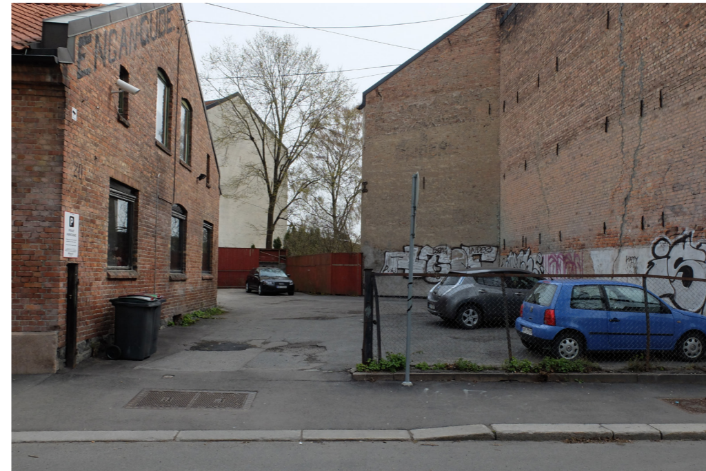
Void between brick building and firewall Akersveien 20
