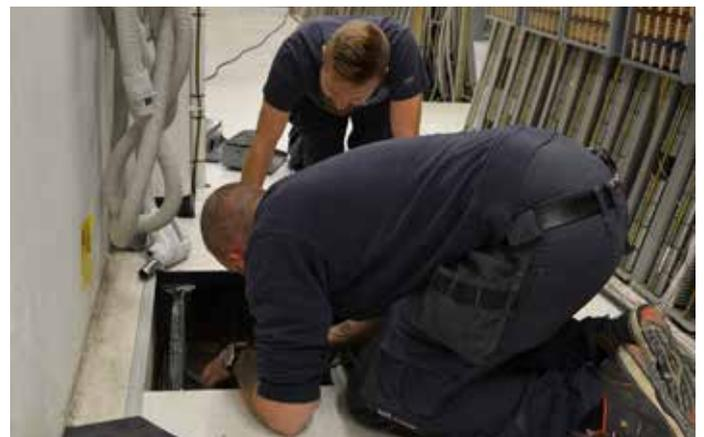
Installing the I-traps among the wiring beneath the floor
