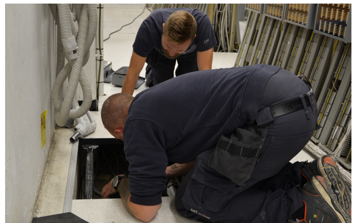
Installing the I-traps among the wiring beneath the floor
