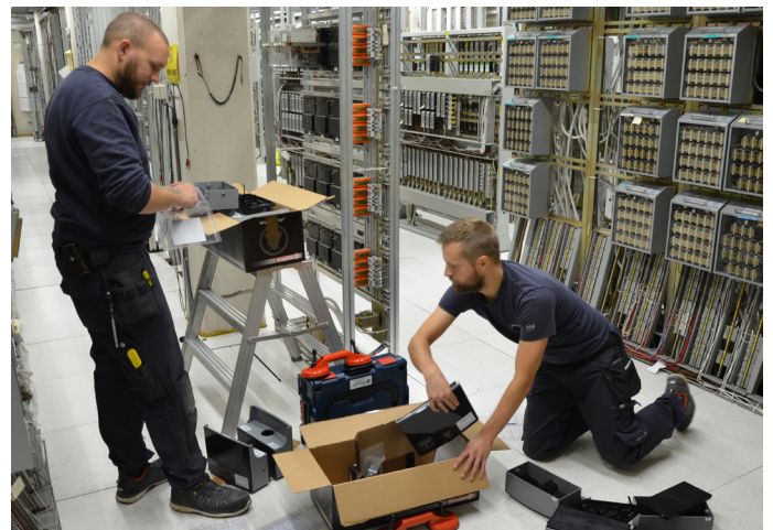
Preparing the I-traps for installation.
