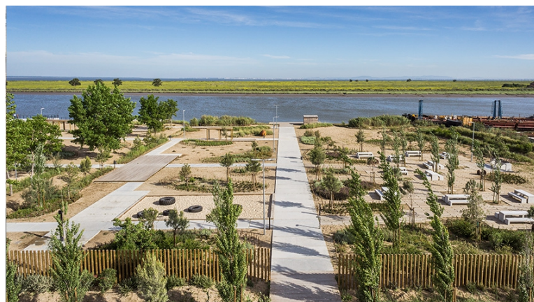
Figure 24: Tagus Linear Park, Portugal, Topiaris, 2013 Attempts at creating inclusive, flexible and multifunctional public space in a 14h regenerated industrial area now providing recreation opportunities by the riverside.
