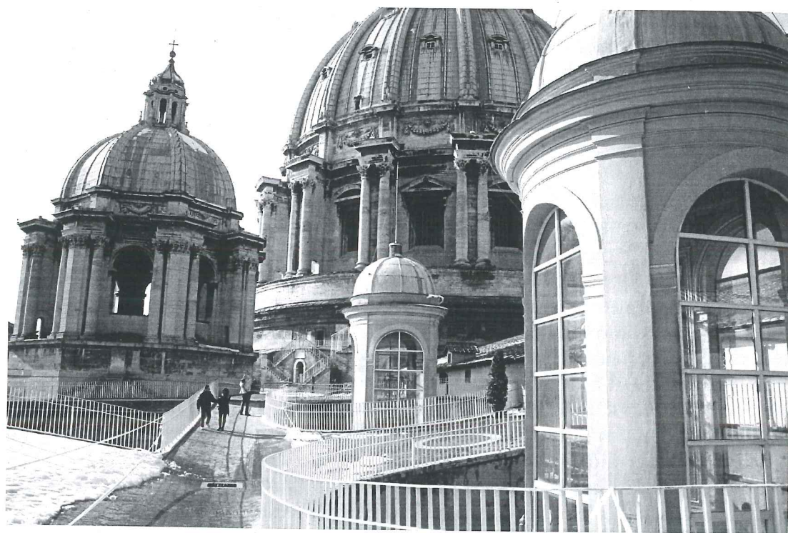
Fig. 1 – The “cityscape” on the roof of St. Peter’s. Author’s photo
