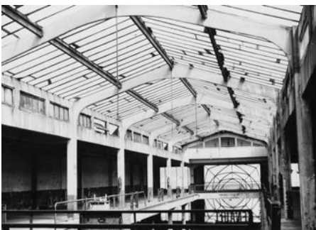
Garage Ponthieu, Paris, by architect Auguste Perret. In 1905 it was one of the first buildings to expose structural concrete.
