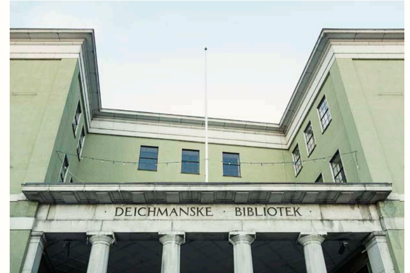
Deichman Library; Skewed facade wall
