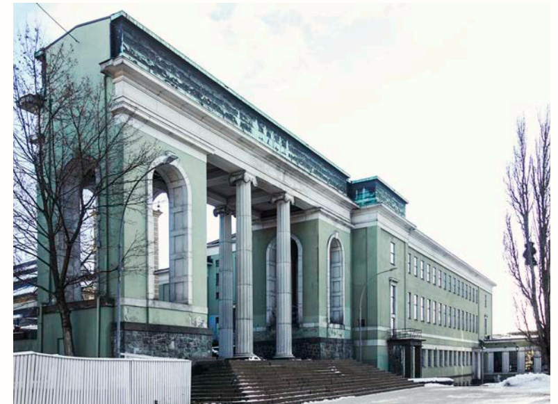
Deichman Library; Rear portal
