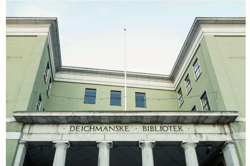
Deichman Library; Skewed facade wall
