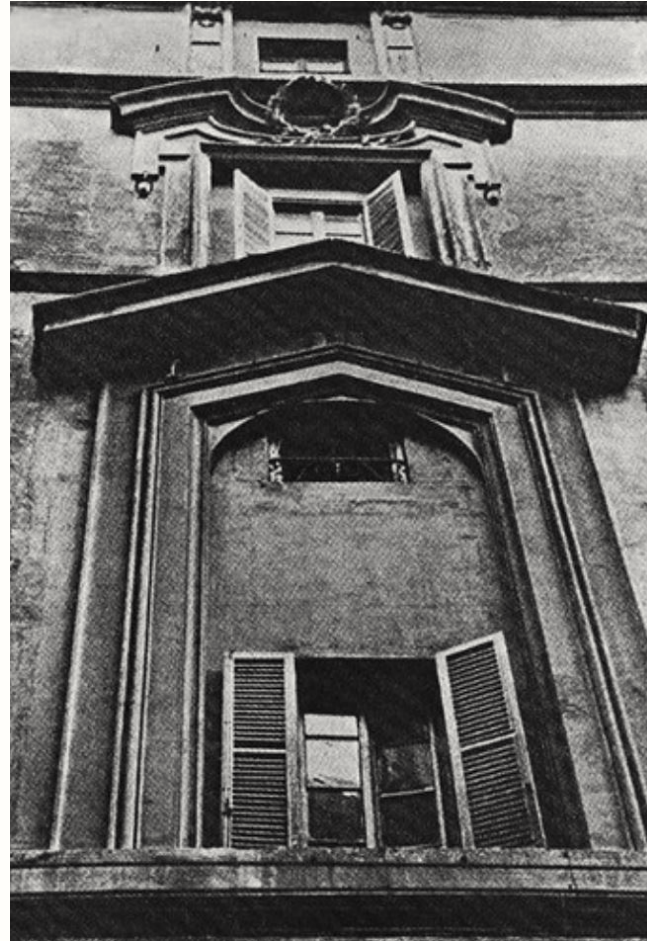
"Borromini's mouldings in the rear facades of the Propaganda Fide are both window frames and pediments."
