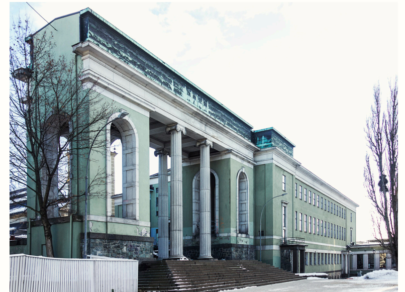
Deichman Library; Rear portal
