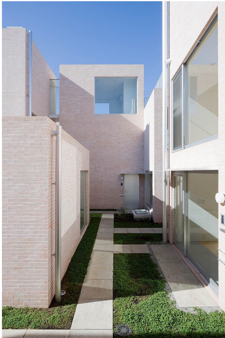
Material: the structure is made by concrete and steel, the other material are brick for the facade, parquet for the floor and aluminum for the windows.
