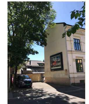
Leftovers in the city structure
