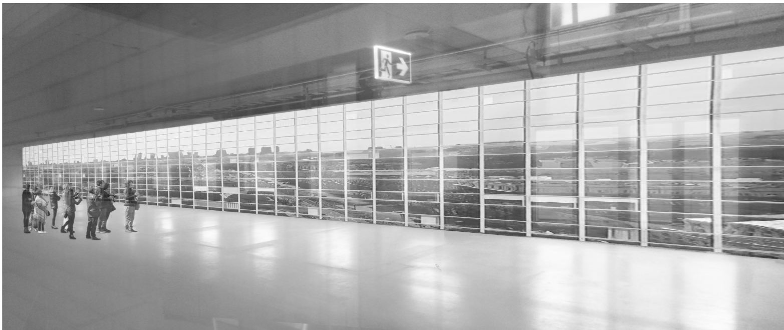
Floor-to-ceiling glass facade
