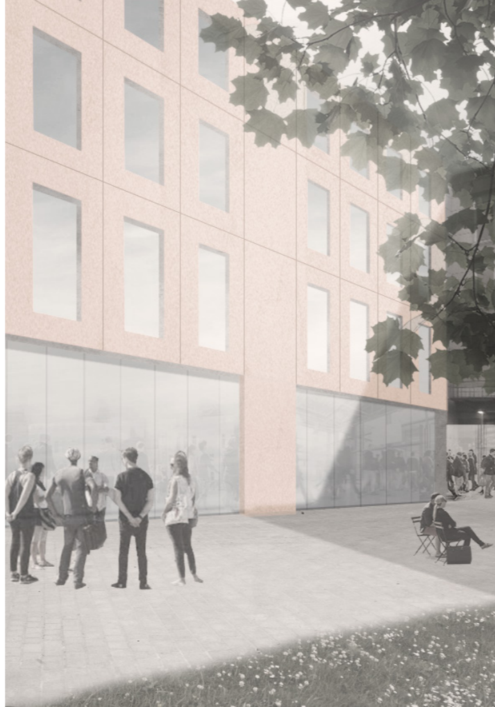
Sand-blasted marble concrete facade elements
