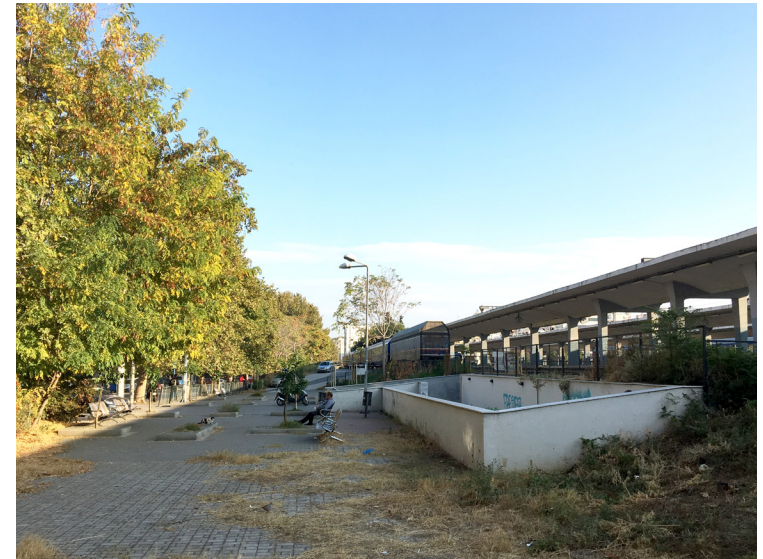
(1) The railway station, entrance facing Xirokrini neighborhood.
