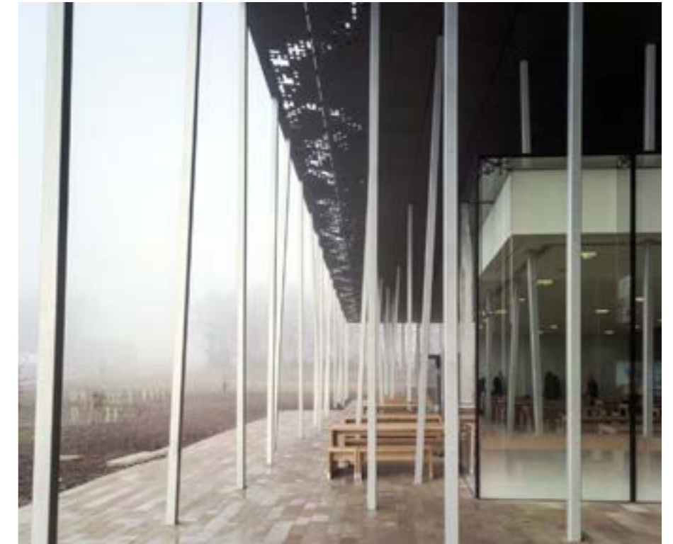
Denton Corker Marshall - Stonehenge Visitor Center: A forest of slender columns creating a filtered spatial environment
