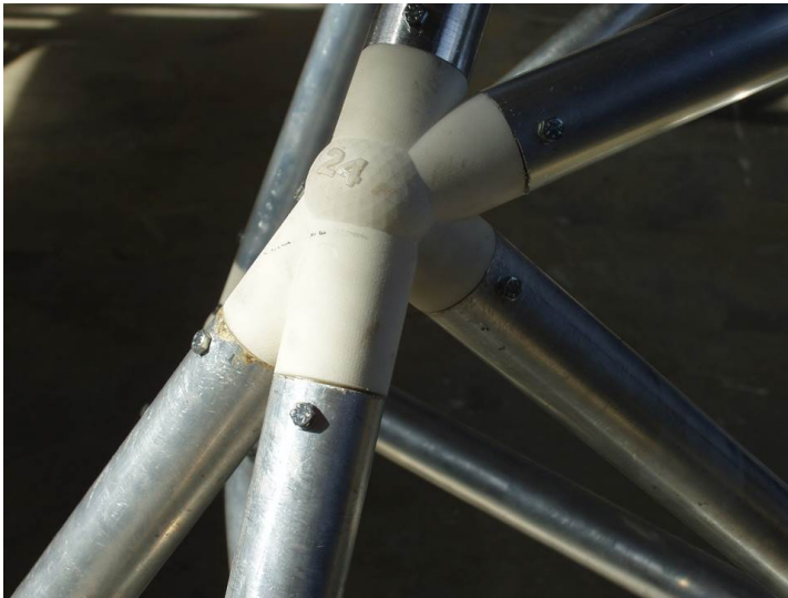
Figure 10 Joint for an architectural installation intended as an entrance gate to a science fair in Oslo. (Design and photo by Espen Bærheim)
