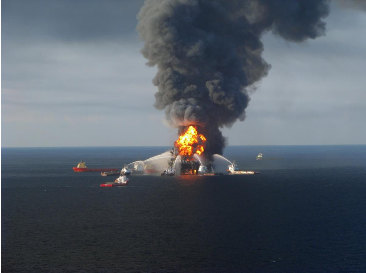
Figure 1. The Deepwater Accident in 2010 and the consequence of poor design. Photo credit: US Coast Guard.
