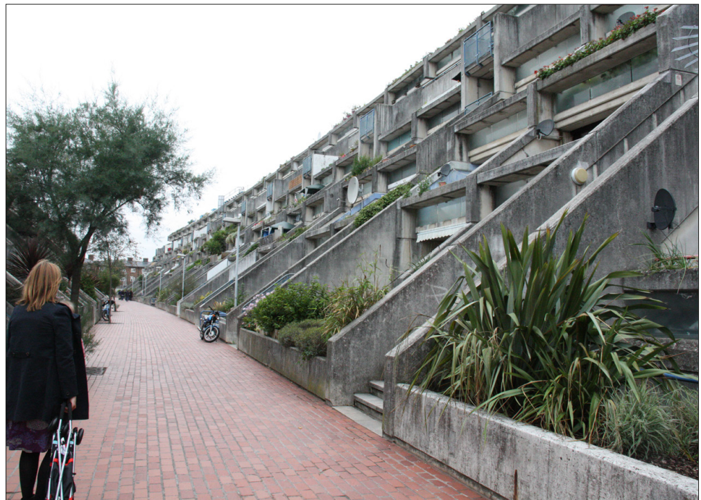
Figure 1. View west along Rowley Way, Alexandra Road. Photo: Tom Davies, 2012
