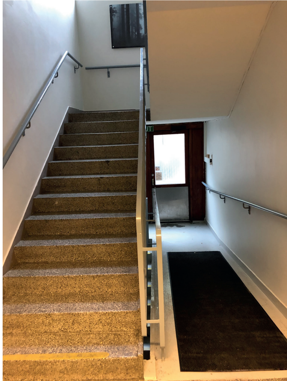
Repetitive staircase cores
