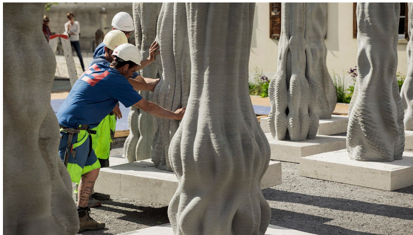
Concrete Choreography - MAS DFAB in Architecture and Digital Fabrication | ETH Zurich
