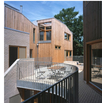
Copper lane, UK http://henleyhalebrown.com/works/copper-lane/
