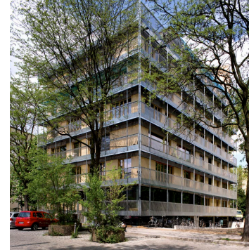
R50 co-housing, Germany https://www.archdaily.com/593154/r50-nil-cohousing-ifau-und-jesko-fezer-heide-and-von-beckerath
