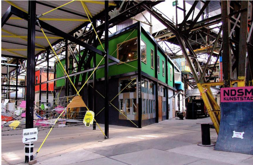
Image 1. The gigantic steel frameworks carrying the colorful DIY fill-ins inside the NDSM hall, designed by Dynamo Architects © Photo: Akbar Simonse
