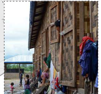
Twin elevated Shelter
