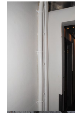
in-situ concrete wall
