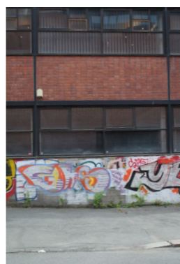
lower vegetation front facade
