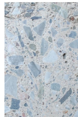
cut concrete in door-frame
