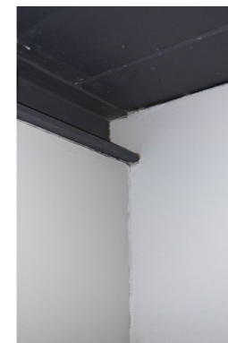
painted steel beam
