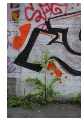
lower vegetation front facade
