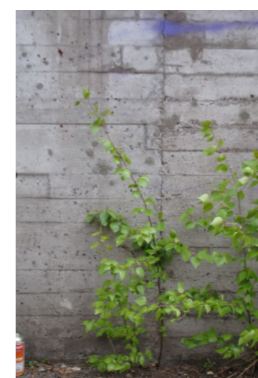
lower vegetation front facade
