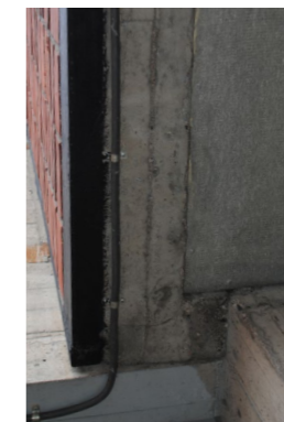
concrete overhanging roof
