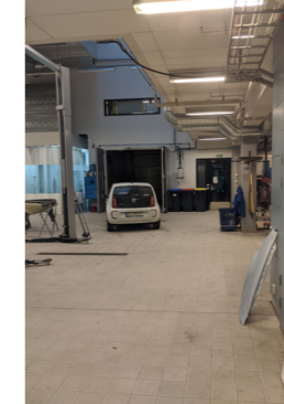
The tiles in the floor are highly un-suitable and not durable. The white colors reveal all damage and dirt
