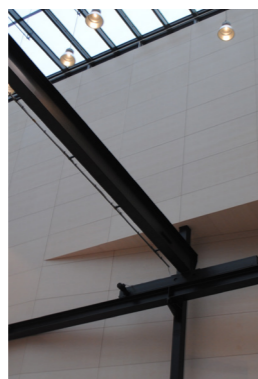
skylight project hall
