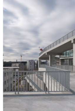
view from roof terrace
