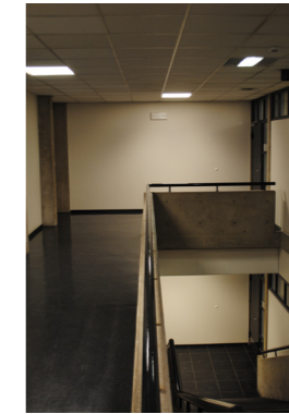
- The stair is situated in the buildings inner areas= no outer windows = the stair-way appears as too dark -low ceiling height
