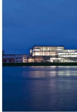
+ the transparent facade let the interior lighting up. A shining lantern by the river that reach attention
