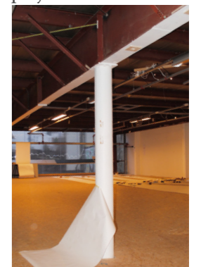
upper mezzanine in project hall
