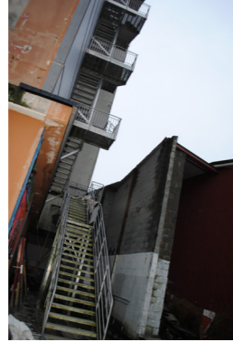
Exterior fire stair
