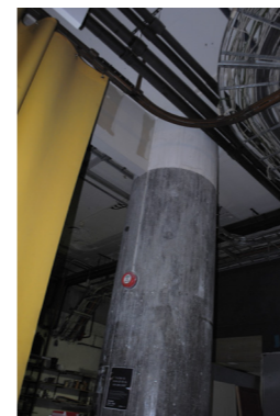
bearing concrete columns
