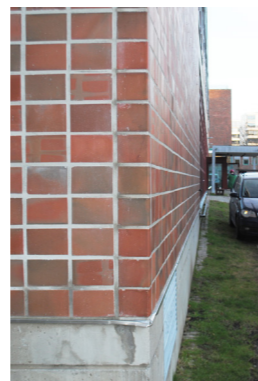
+ The terracotta tiles are in good condition
