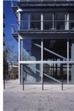
+ transparent and open facade towards the street. show the daily activity in the school
