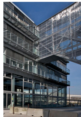
+ industrial and rough materiality that is suit the program and is cheap: corrugated polycarbonate, glass, concrete and steel.
