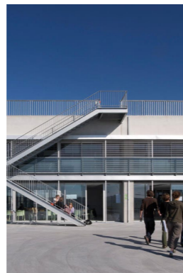
+ a large public roof terrace that offers a great view. the main outdoor area of the school.
