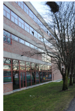
Large windows in some lower parts of the facade. Despite this the building lack a natural transition between interior and exterior spaces.
