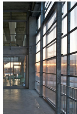
+ the facade mainly consist of large sliding doors that can be fully open= offers a good transition between the interior and exterior spaces.
