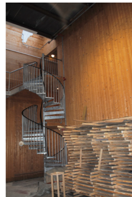
Spiral stair in building hall
