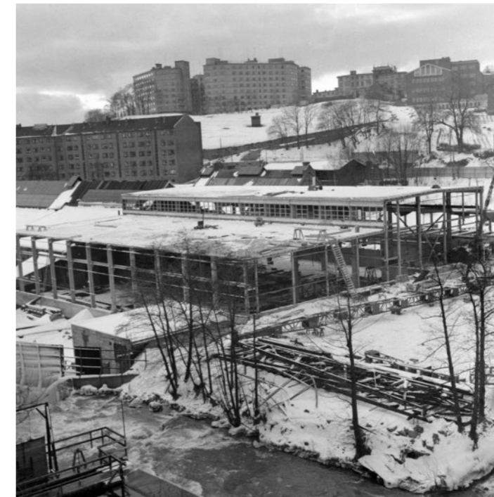
Pictue taken in 1930 during the construction of the new production facilities for "Vulkan", north of Brenneriveien
