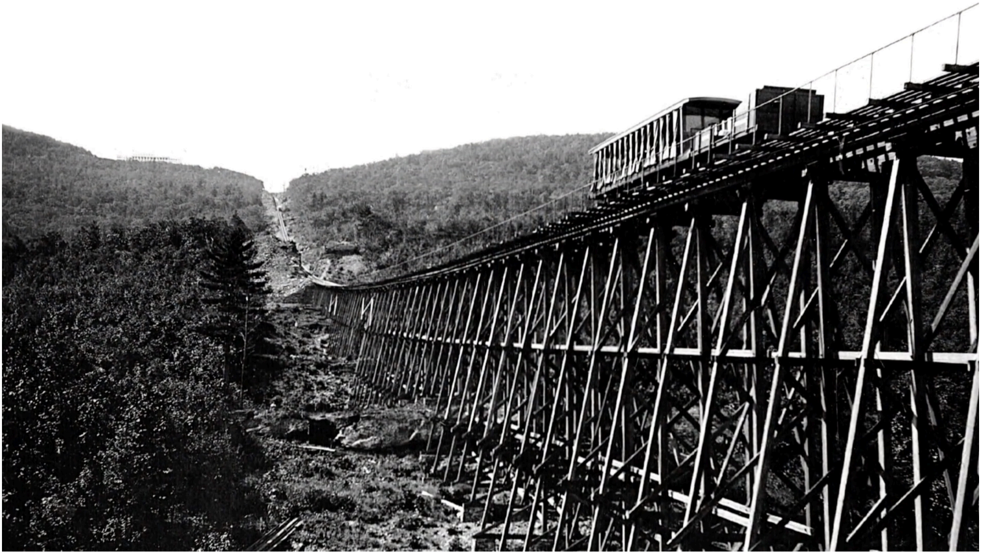
6.17 The elevated tracks of the Otis Elevating Railway. The train was made up of four cars; two for passengers (75-90 people) and two baggage cars.
