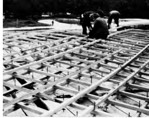
Figure 114 Frei Otto, Carlfried Mutschler and Partners, 1975, Multihalle Mannheim . The laths are laid flat.
