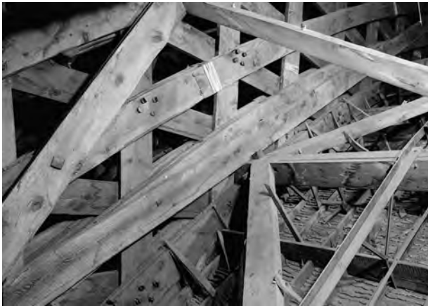
Figure 27 Henry Grow and William H. Folsom, 1864-1867, The Mormon Tabernacle at Salt Lake City. Jointing made by wooden pegs and cowhide lashing.
