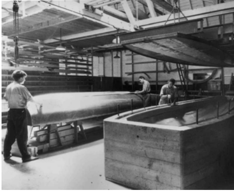
Figure 40 Forming Loughhead monocoques in concrete moulds.
