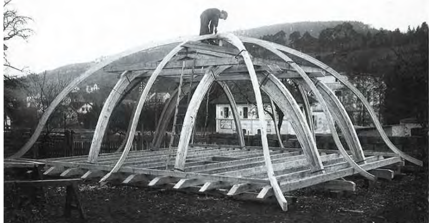
Figure 112 Hetzer AG, 1910, crematorium curved glulam timber roof structure, Baden-Baden.
