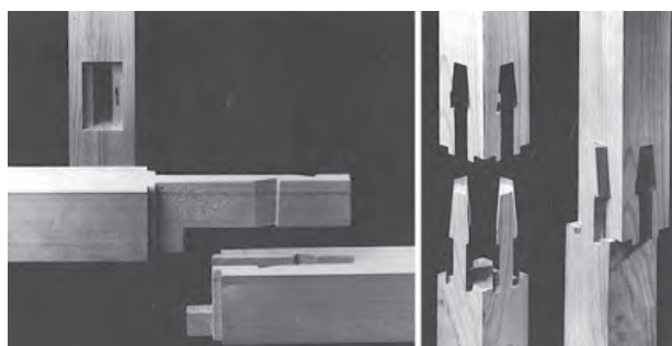
Figure 1. Tsugite – Japanese splicing joints (image source: [1])
