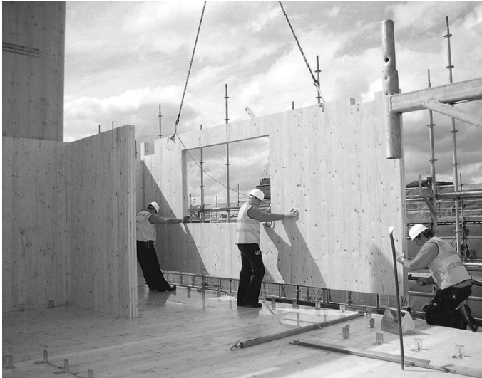
Figure 84 Hugh Strange, 2014, Architecture Archive, Somerset, installation of exterior CLT walls.
