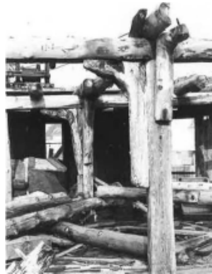
Figure 52 Norwegian bent construction or cross frame ( grindverk ).
