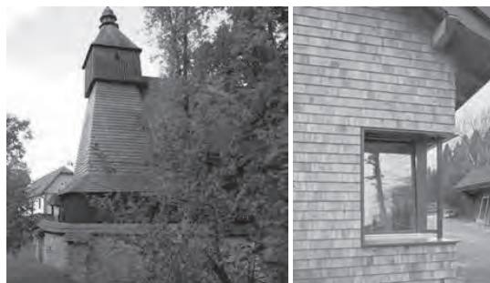
Figure 17. 16 th century church in Hervartov (Slovakia) made from yew (photo M. Wójcik) and 2013 Albisgüetli forestry operations centre in Zurich clad with yew shingles (photo H.Henz, source [43])
