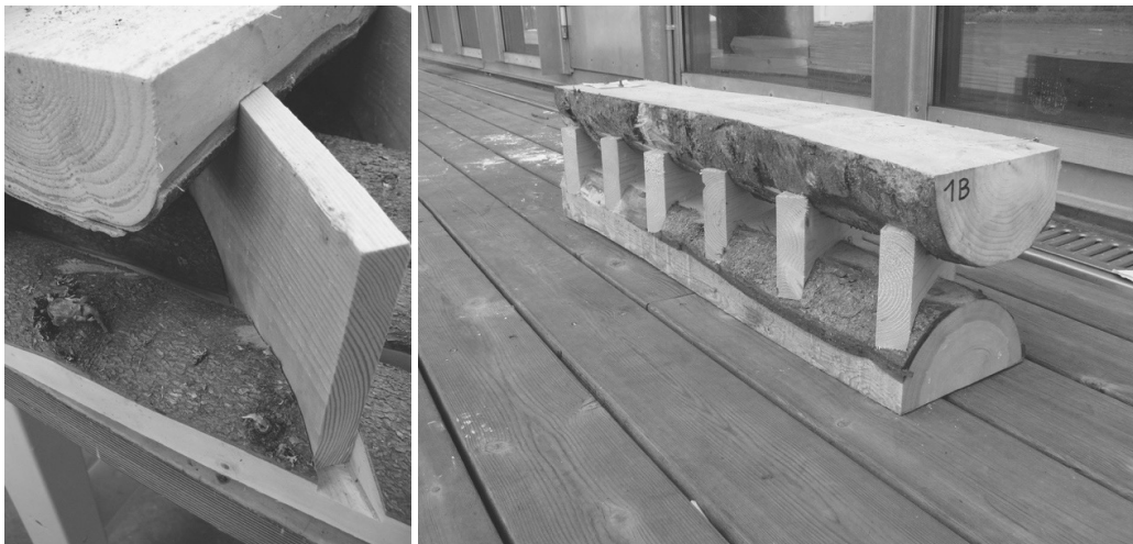
Figure 33 BackToBack , dry-in-wet . Left: Connection detail. Right: A series of dry pine boards inserted into parallel incisions .
