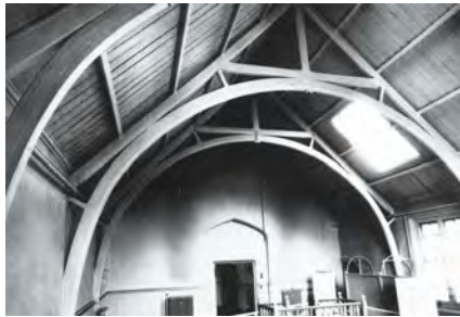
Figure 109 Assembly hall of King Edward College, Southampton, 1860.
