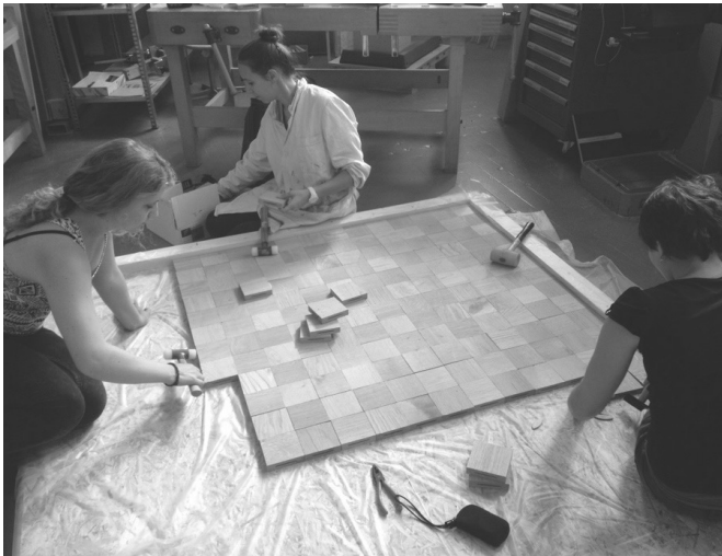
Figure 45 The Swelling Vault , laying the parquet blocks.
