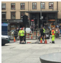
Construction and renovation
