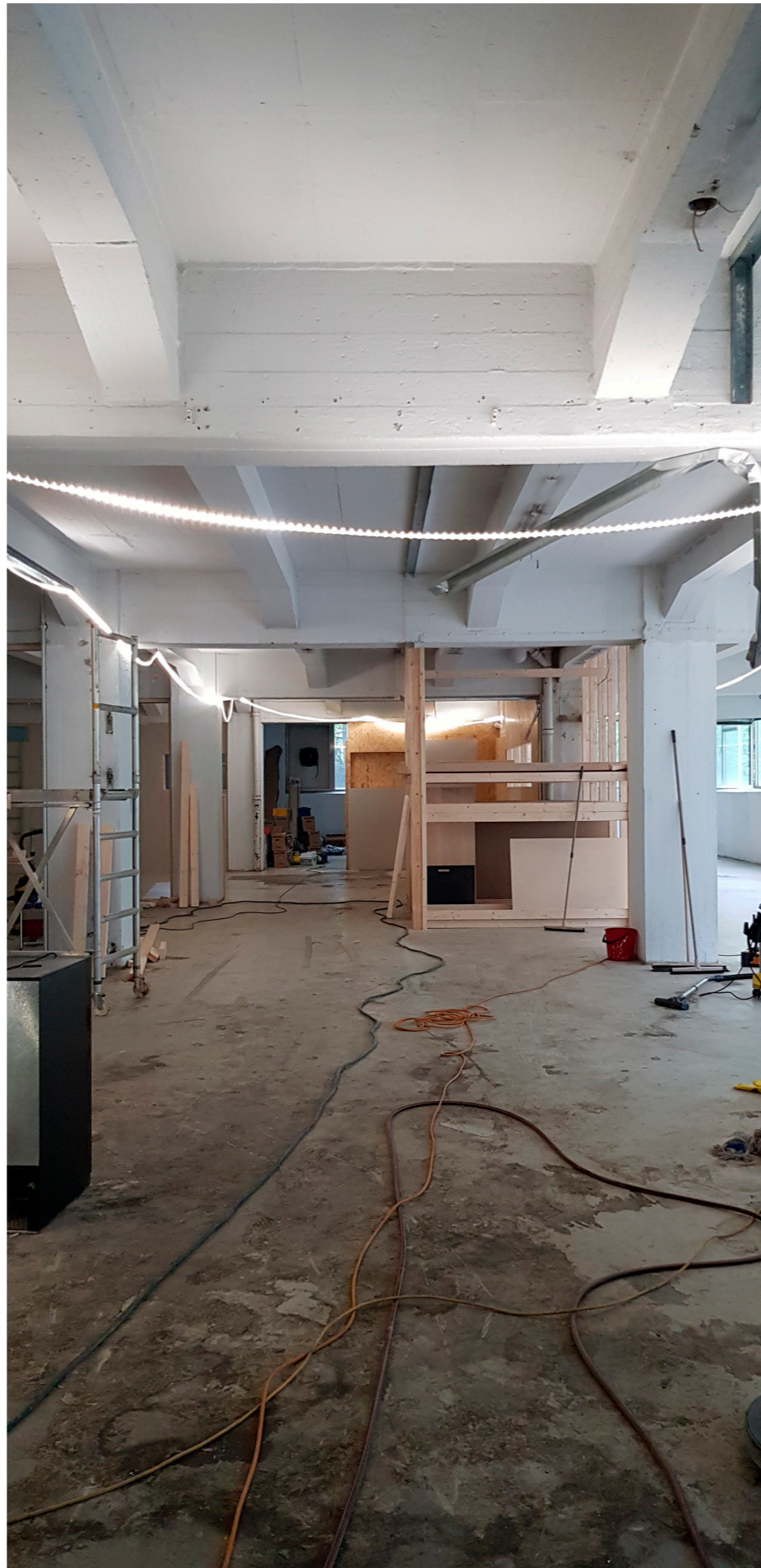
Concrete skeleton grid, U2 floor
