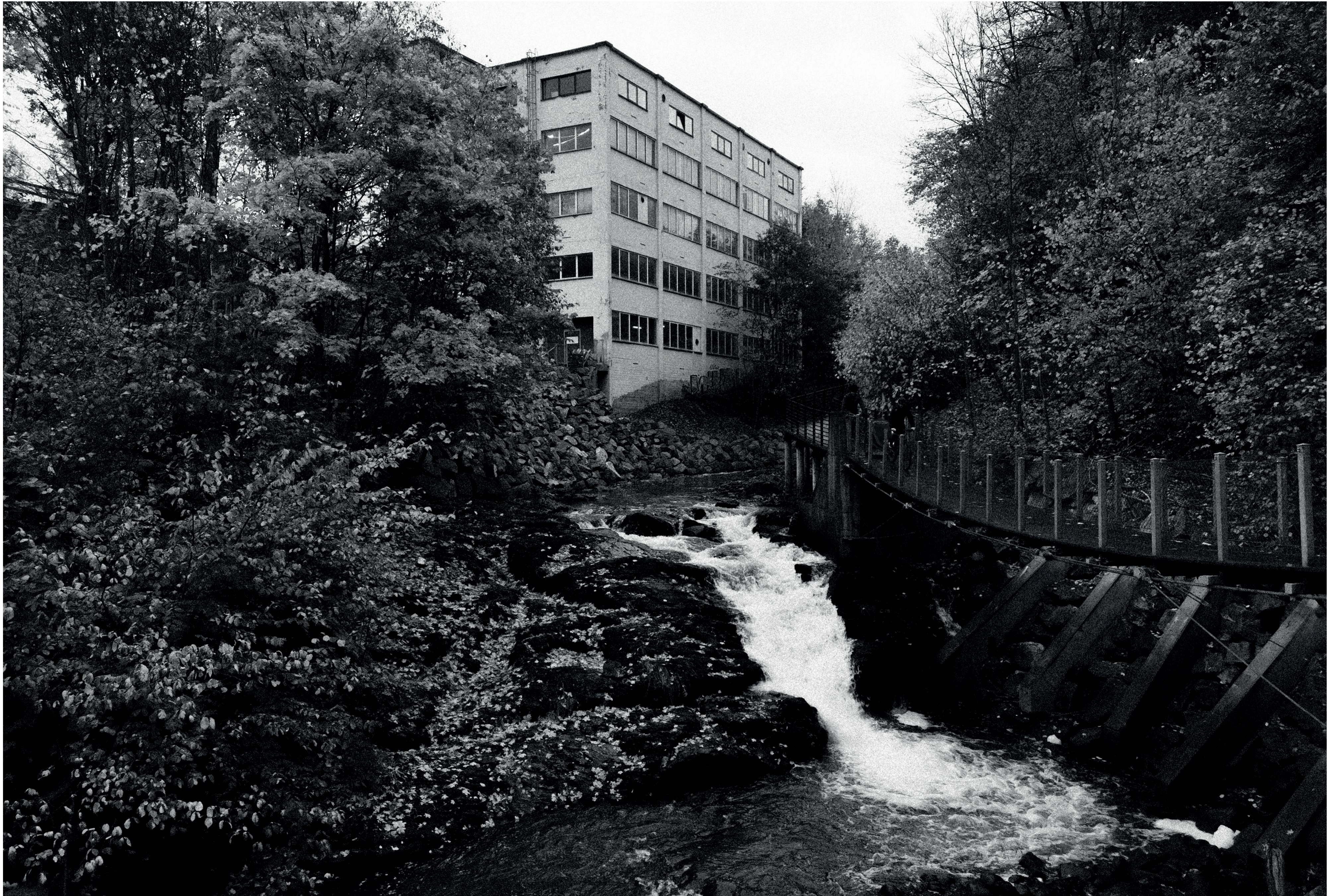
Existing situation and structure
