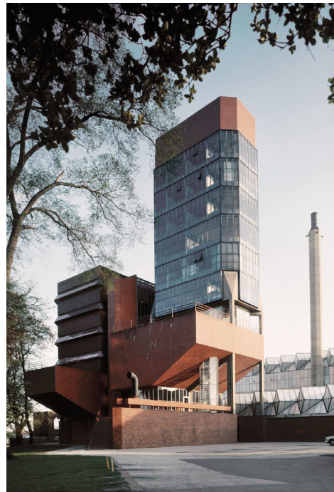
Leicester Engineering Building; Stirling & Gowan 1960
