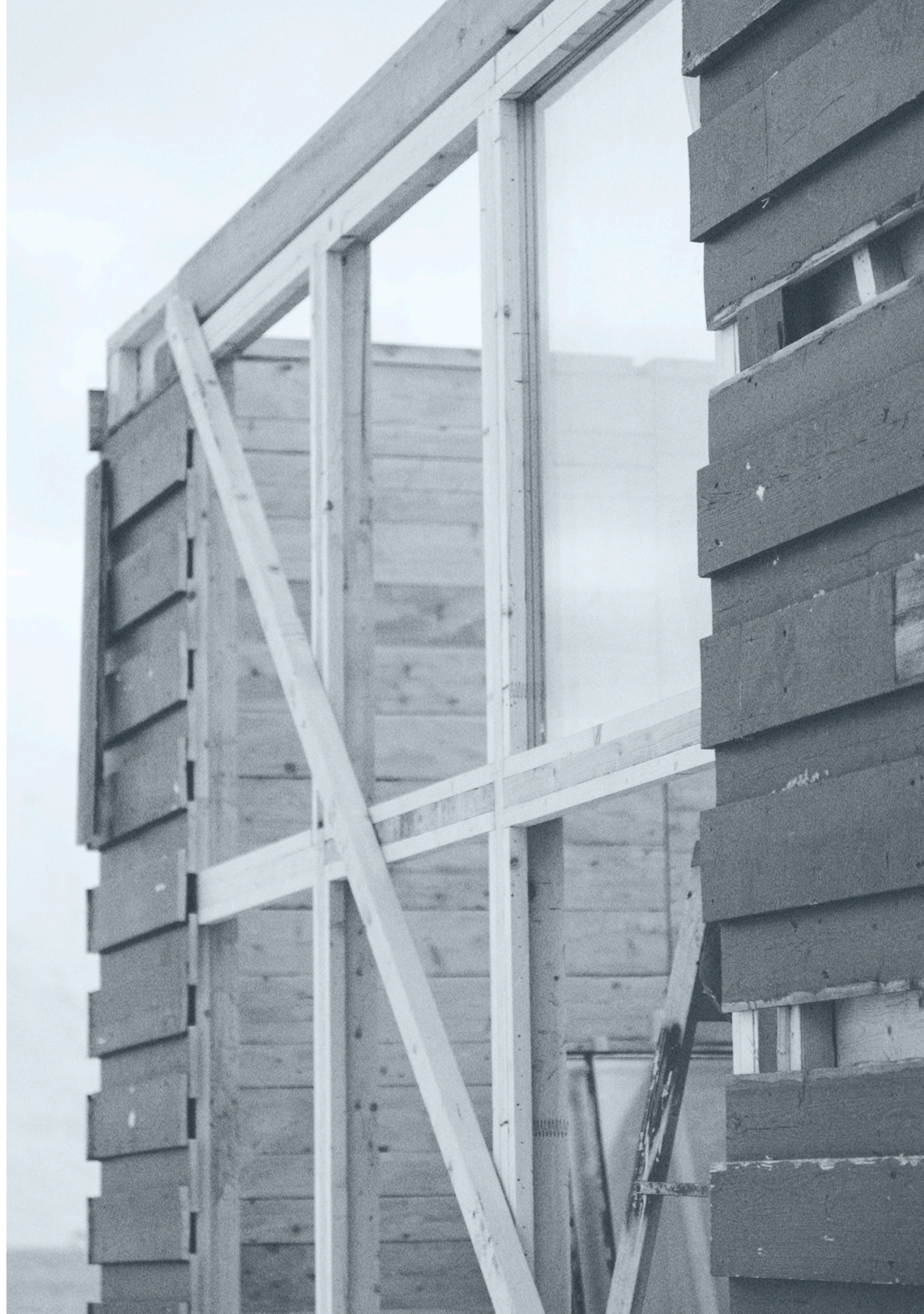
07. In Feb 2020, the author was involved in a student-led project tasked with designing and building a sauna in Longyearbyen, Svalbard. The structure was constructed entirely from reused wooden studs and cladding. Panes of glass from reclaimed windows were removed from their frames and incorporated in (re)new floor-to-ceiling glazing.
