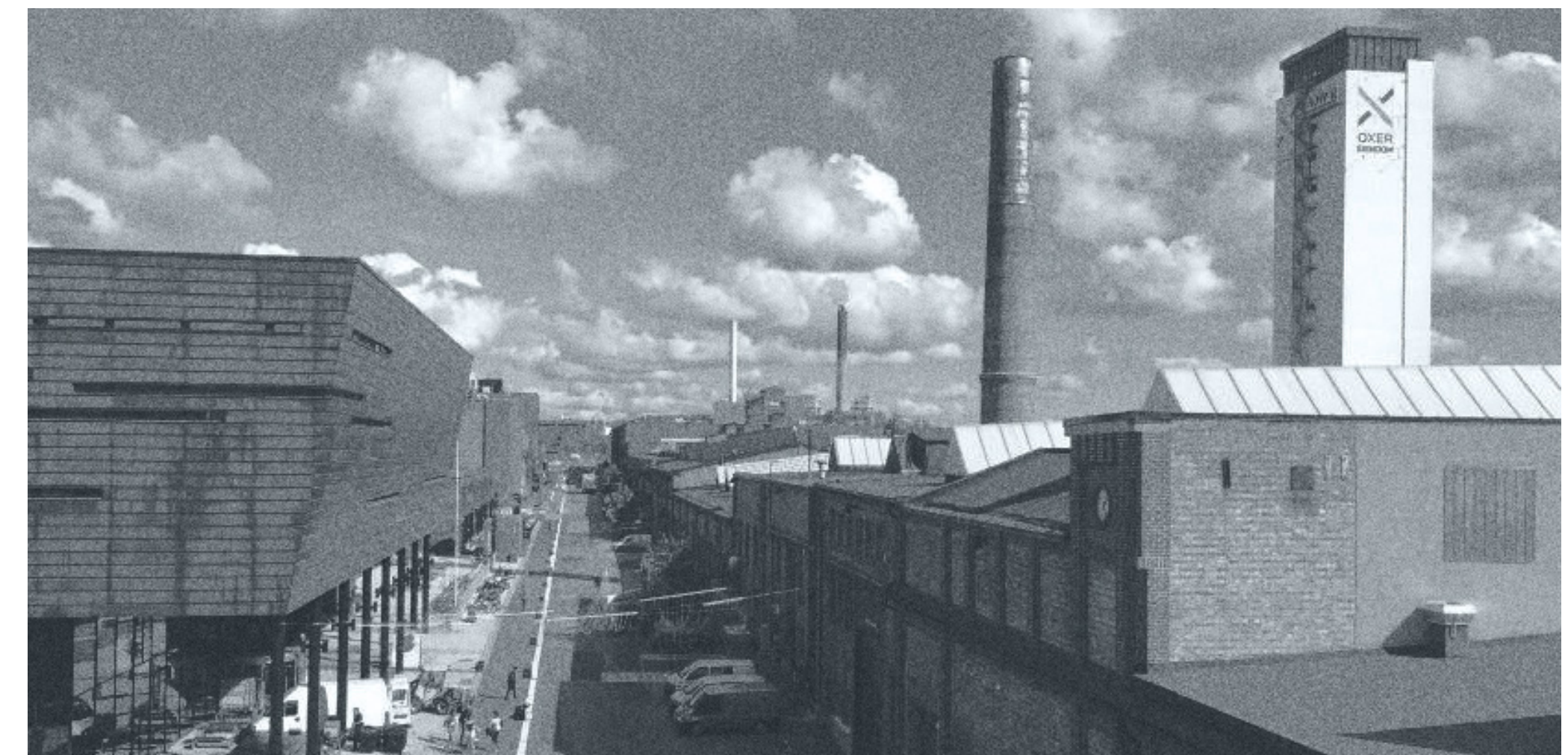
11. Kabelgata. To the left is the vocational school. The right, the defunct cable factory, now home to numerous other businesses. It is protected under historical heritage bylaws.
