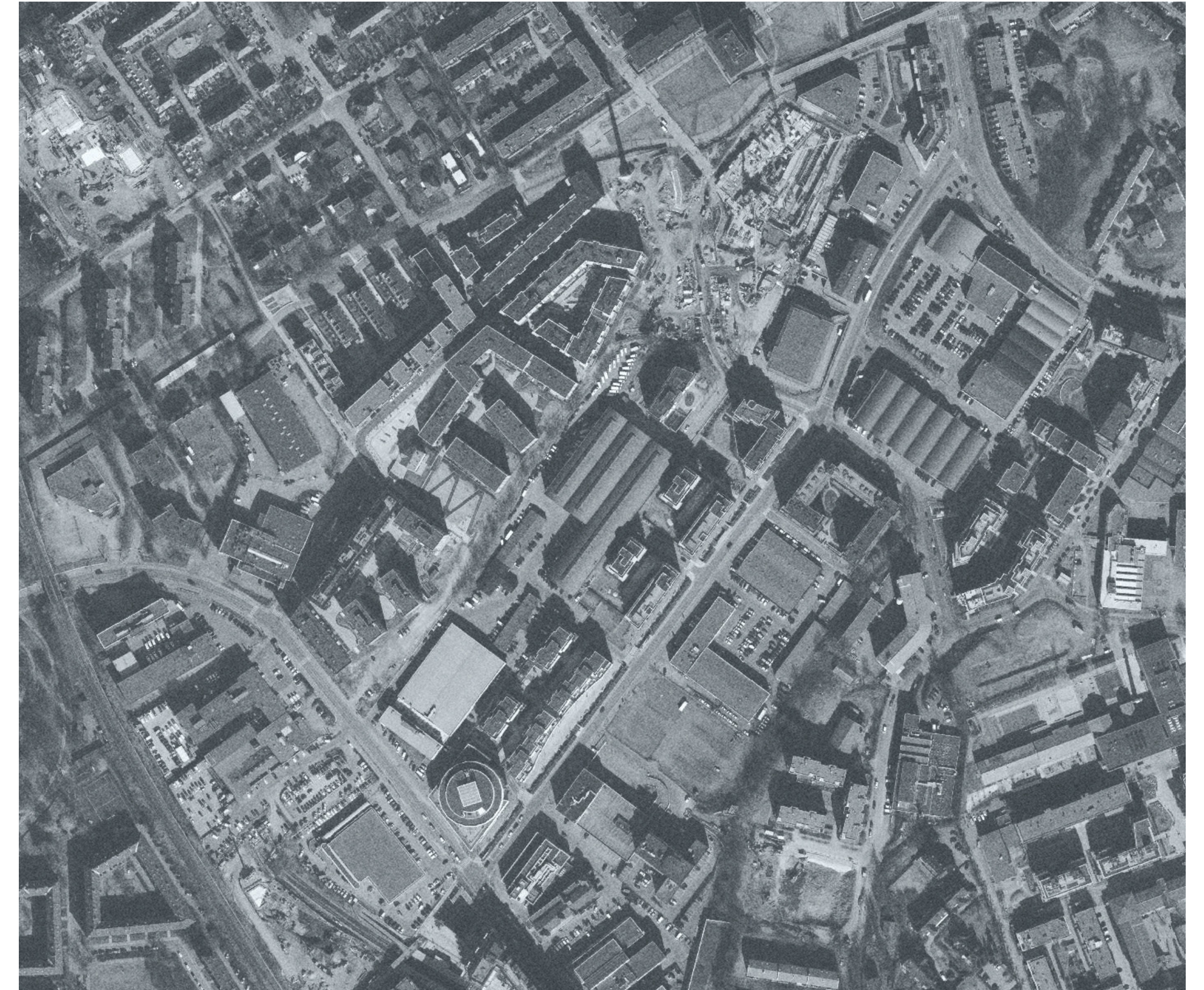
09. A changing context, Gladengveien 8 in 2020. Two of the five halls have been removed, although it is unclear exactly when. Ensjø along with the rest of Hovinbyen shifts away from the industrial past. Apartment blocks are clearly visible here, changing the urban fabric. Most if not all of the remaining industrial buildings will be gone in the next 10-20 years.
